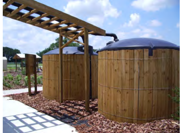
A rainwater harvesting cistern used for irrigation.
