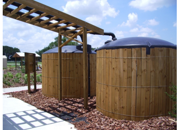
A rainwater harvesting cistern used for irrigation.
