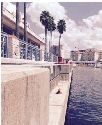
The Seawall has proper bollards and cleats installed to accommodate docking.
