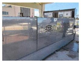
sludge with a 7% t solids concentration. The remainder of the wasted sludge flow (average of 15 gpm) bypasses the RDT and flows directly into the sludge holding tanks. This waste activated sludge flow, with a solid's concentration of 0.5 - 0.7% percent is used to dilute the thickened sludge. The target sludge holding tank solids concentration is 2.5 - 3.0% solids.
