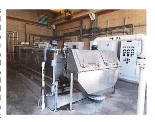
• **Dewatering** - Dewatering of bio-solids is accomplished by pumping anaerobic digested sludge from the GSH tank to feed one, two, or three dewatering centrifuges at a variable feed rate of 4% - 5% solids concentration. Dry micro-bead polymer is injected through a
