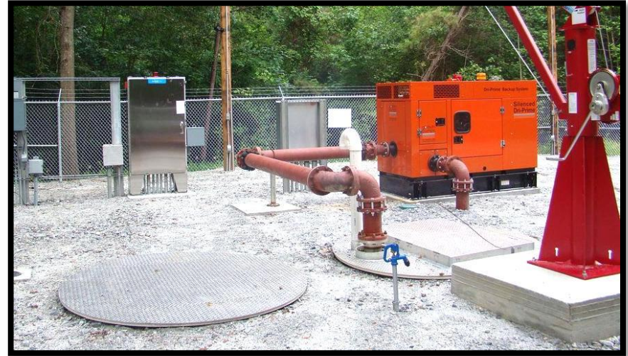
Diesel powered bypass pump
