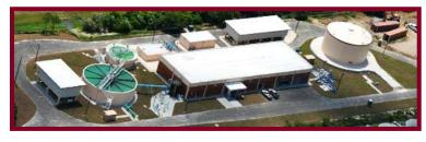
The WTE Facility requires a large amount of water for the cooling towers to cool hot steam made in the WTE Facility after it exits the turbine generator. Solid Waste built an Industrial Water Treatment Facility that can provide all the necessary water by taking water from a
