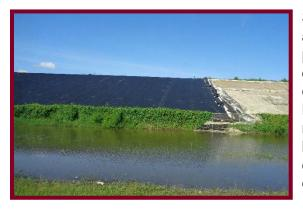
Solid Waste created the landfill by forming clay walls around the Earth's natural clay layer underground to provide a resting place for waste. When Solid Waste dumps trash in the landfill, it spreads, crushes, and covers the garbage with ash from the WTE Facility. Because there is limited landfill space, Solid Waste makes every attempt to bury only waste that cannot be burned or recycled, such as boats, mattresses, couches, construction debris, and large items of commercial waste.
