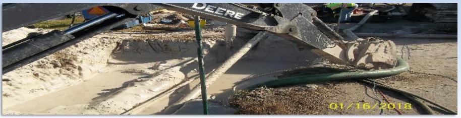
**Description:** Construction of a new 24" force main with conversion of original for use as a redundant main for back-up.
