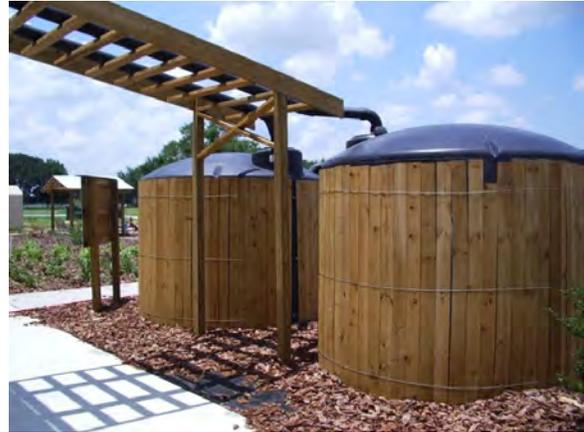
*A rainwater harvesting cistern used for irrigation.*
