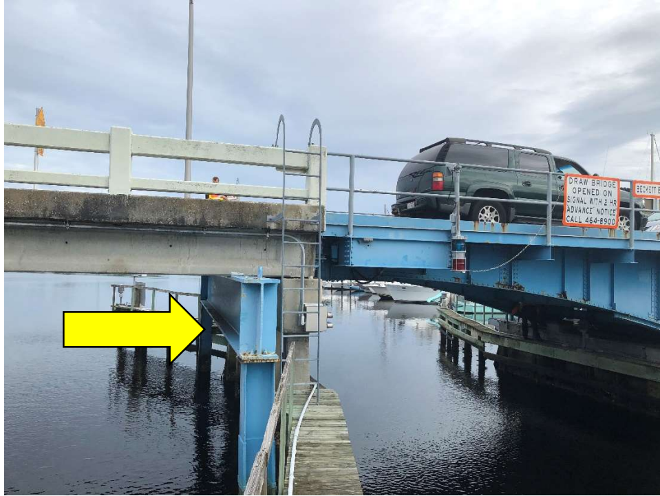
Photo 3 - Crutch Bent at Rest Pier/Bent 6
