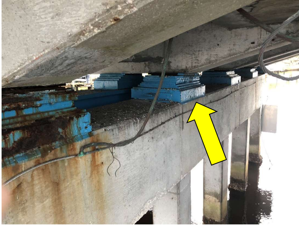
Photo 7 - Shims/Blocking at Bent 7 to Address Prior Settlement
