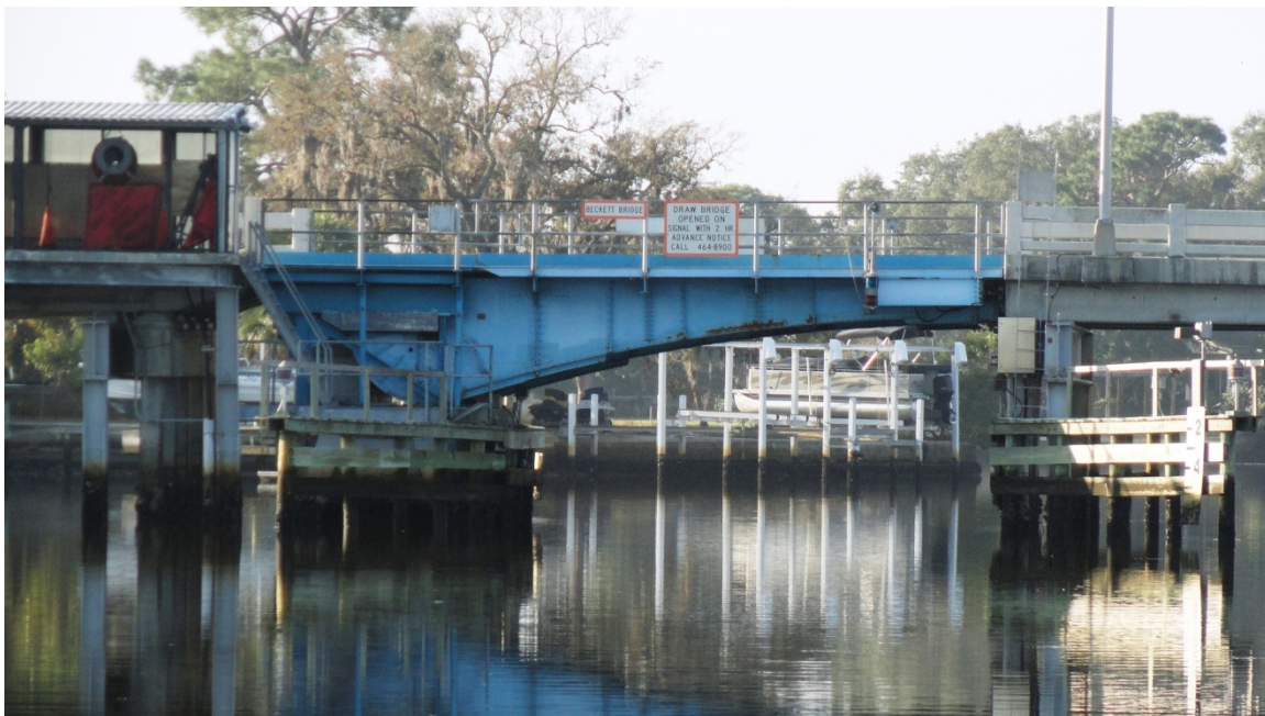
Bascule Leaf in Closed Position
