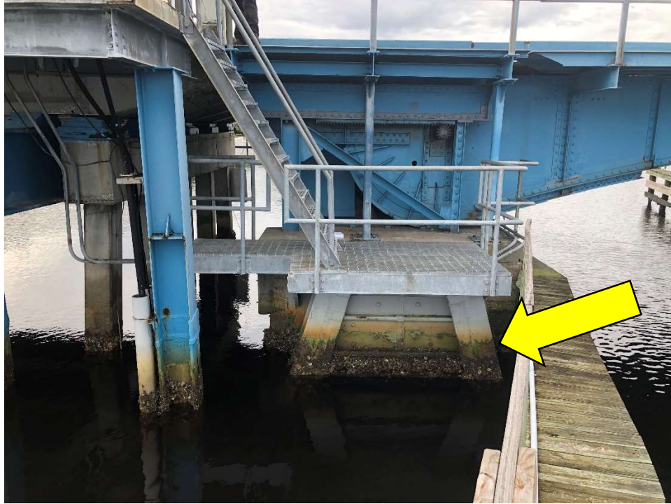
Photo 8 - Bascule Pier Helper Piles at North Side
