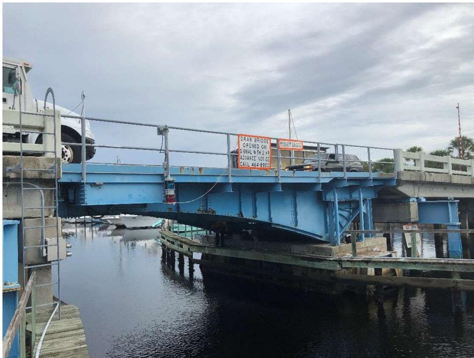
Photo 4 - Bascule Span
