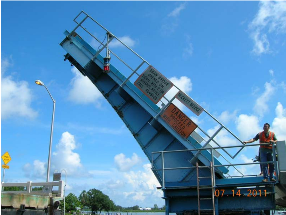
Bascule Leaf in Full Open Position
