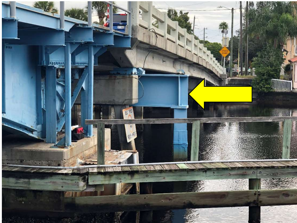
Photo 6 - Crutch Bent at Bent 7
