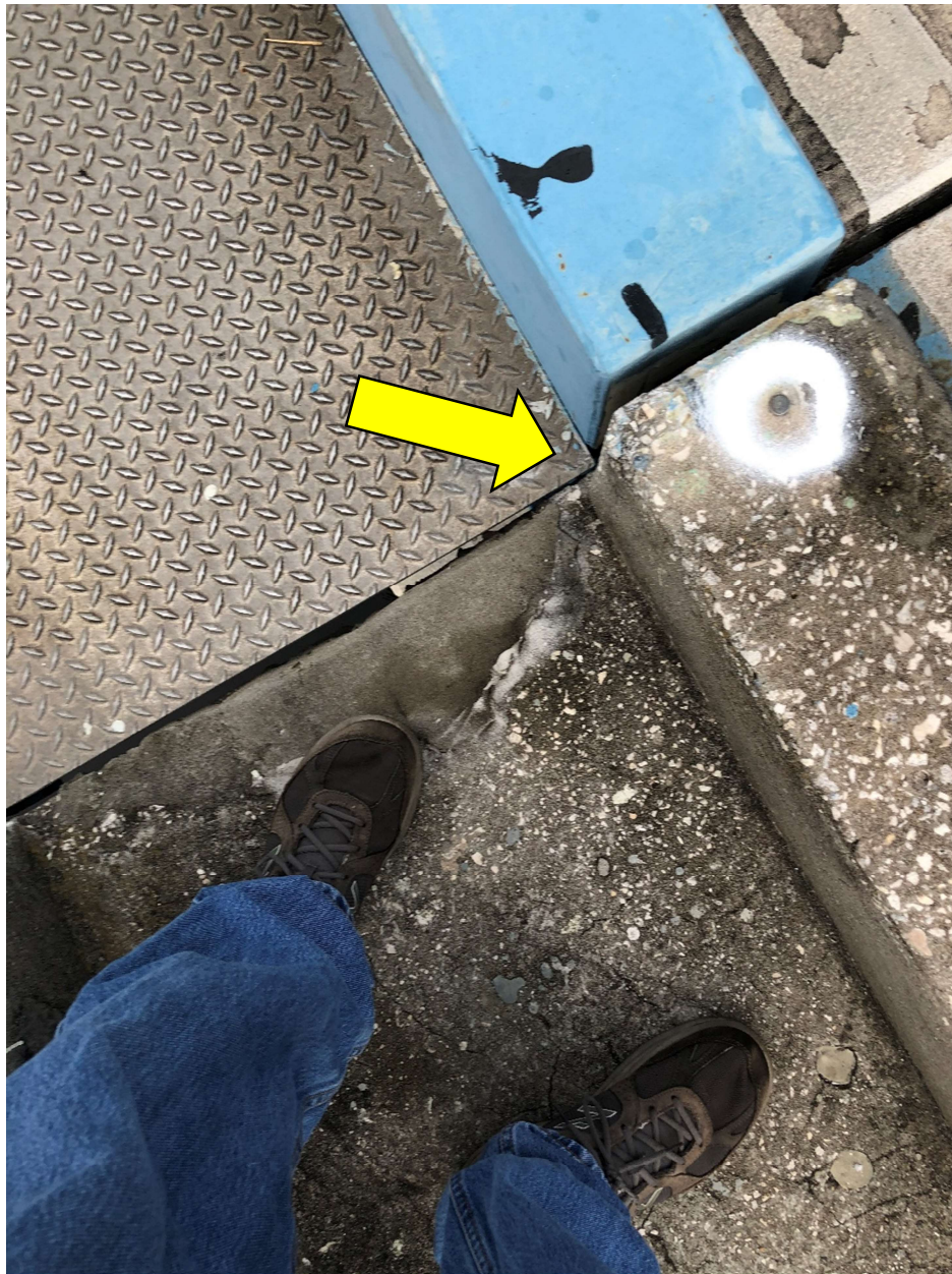
Photo 14 Sidewalk Joint at Bascule Span with Evidence of Horizontal & Longitudinal Movement/Rotation
