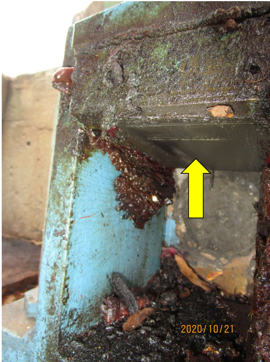
Photo 16 - Span Lock Receiver with Evidence of Tight Contact with Lock Bar from Rest Pier Settlement
