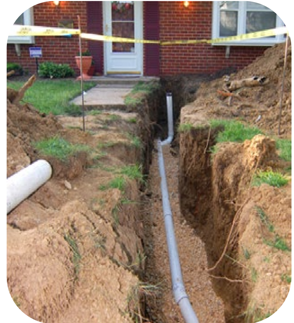
Private Sewer Lateral Construction
