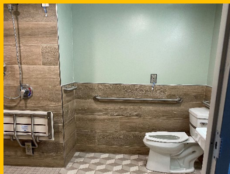
PARC Bert Muller Facility Improvements - Bathroom Renovations Phase 1
