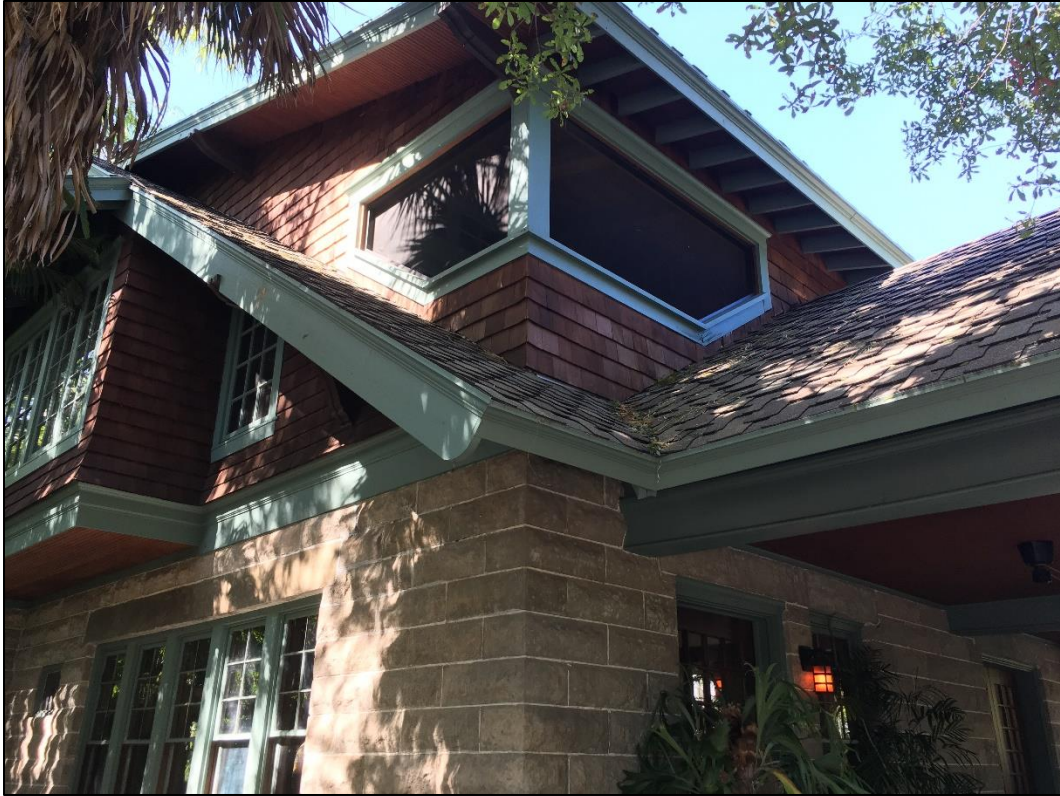
Figure 11: Sleeping porch dormer alteration, post-construction
