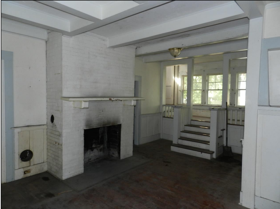
Figure 5: Interior room with fireplace and stairs, prior to construction
