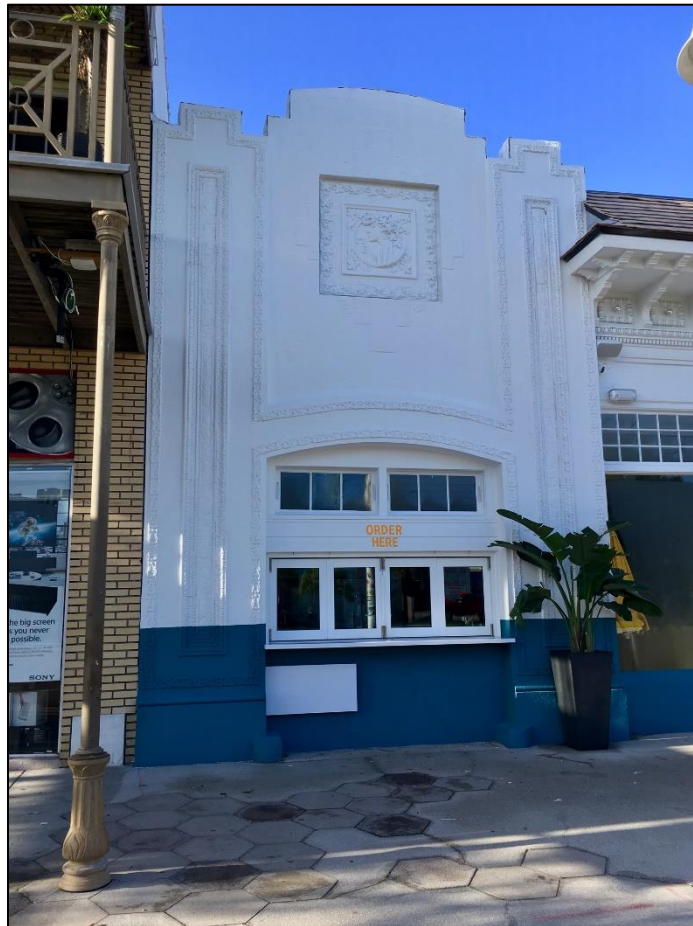
Figure 2: Detail of new takeout window and stucco repair
