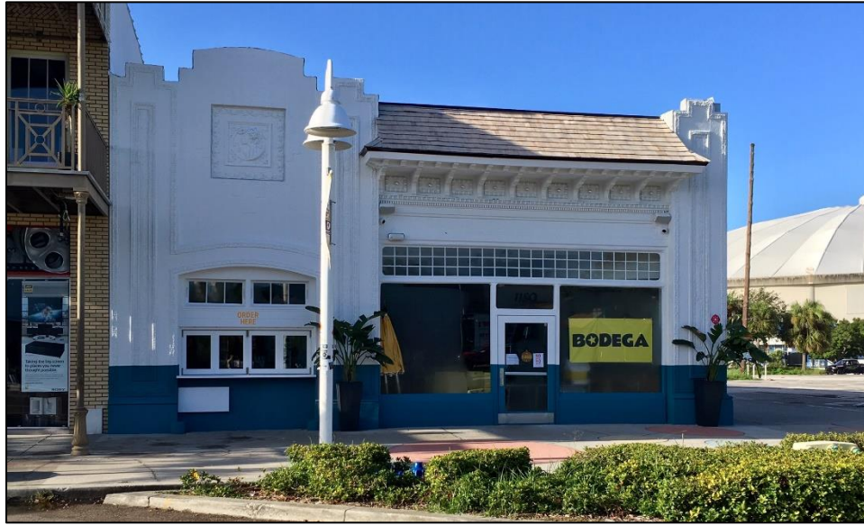
Figure 1: Front façade of subject property, post-construction
