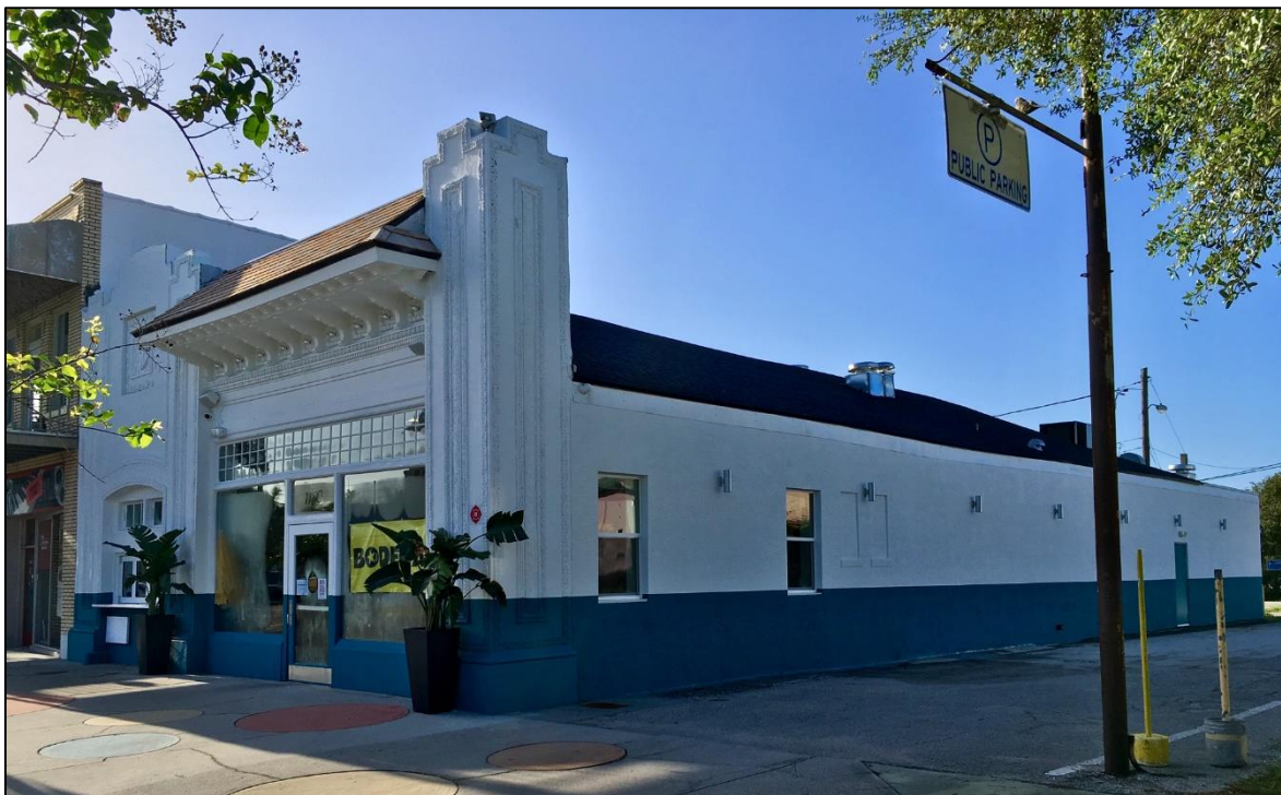
Figure 4: Front and side façade
