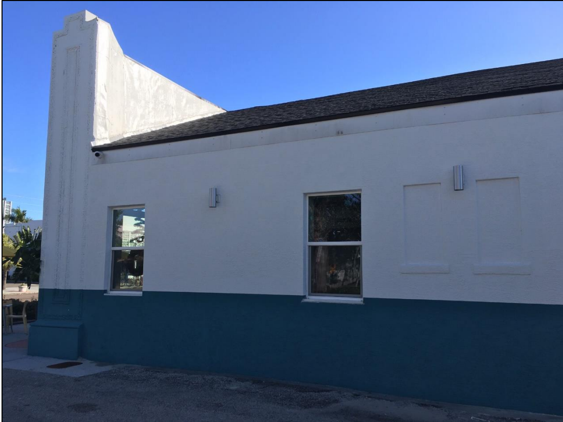
Figure 5: New windows and new asphalt shingle roof
