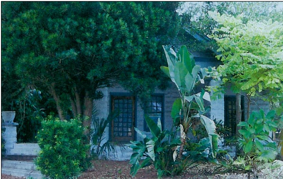
Figure 2: Front façade prior to construction
