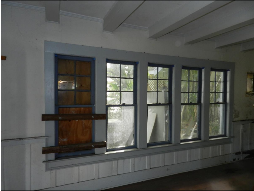
Figure 7: Windows prior to renovation
