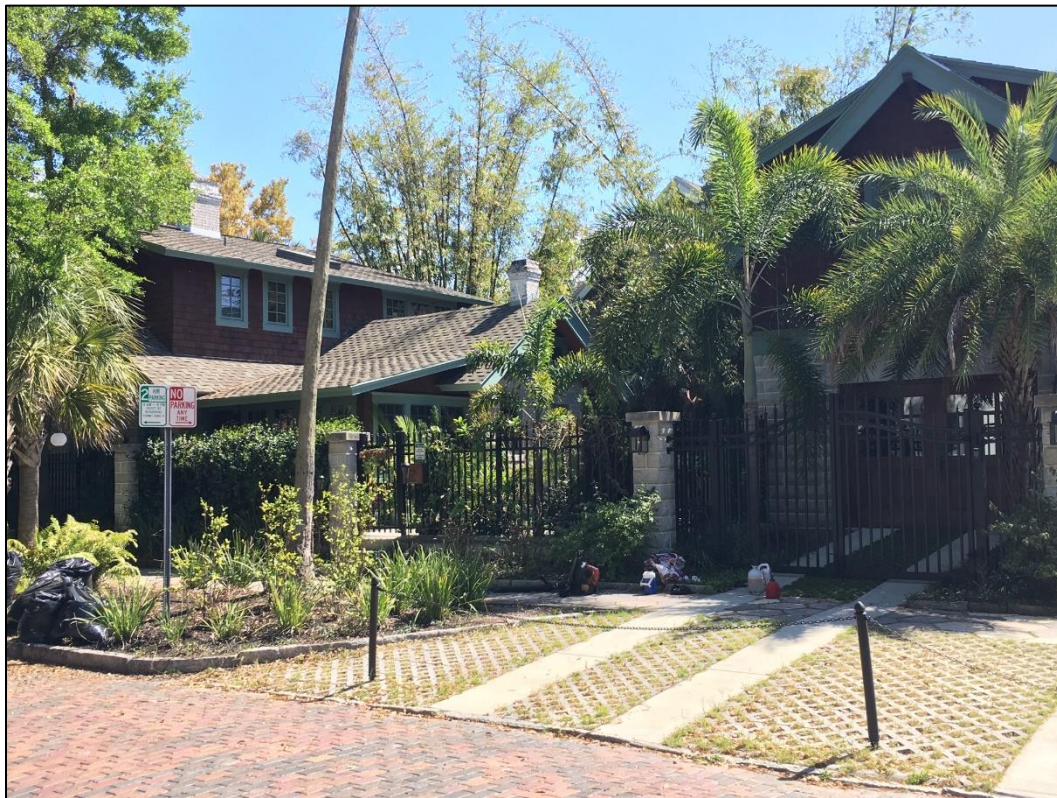
Figure 18: New garage and rear of house, post-construction
