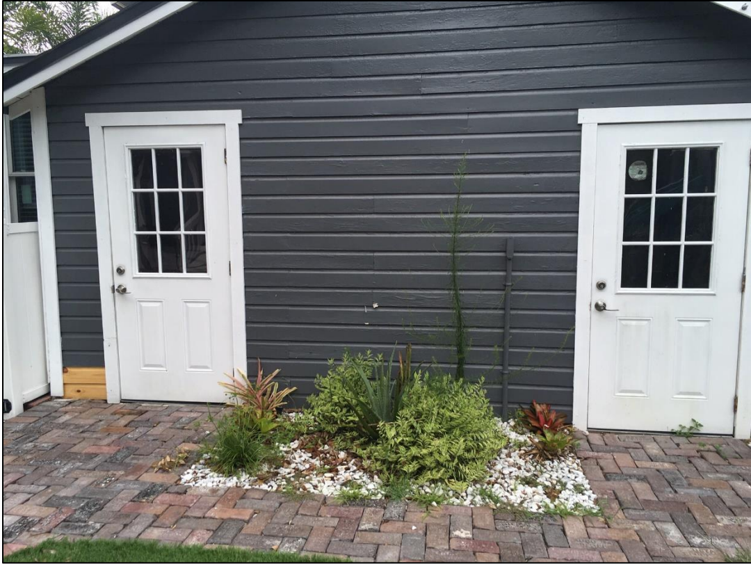
Figure 5: Garage after structural repairs and HVAC upgrade
