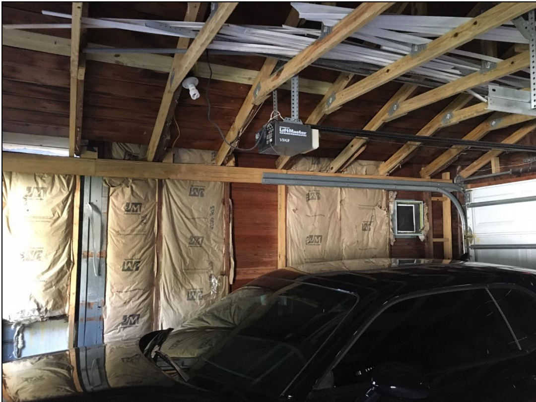
Figure 6: Garage after structural repairs and HVAC upgrade
