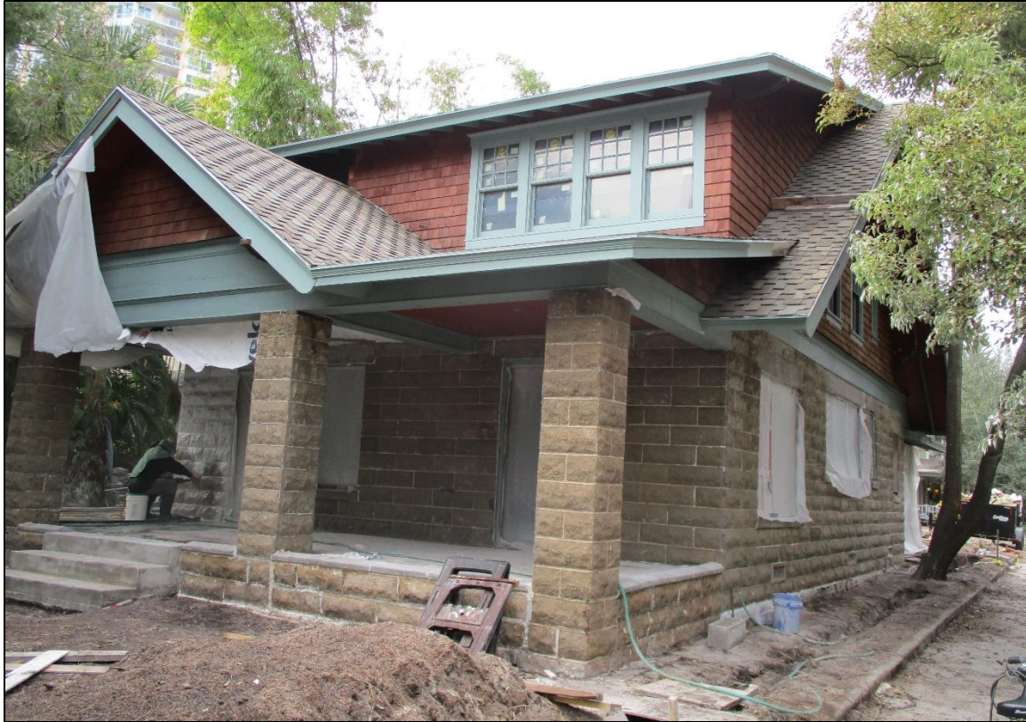
Figure 3: Front of property during construction
