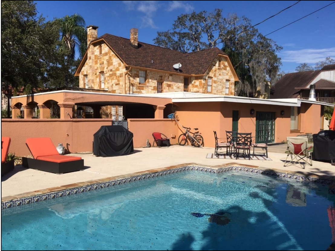
Figure 7: Rear of house, showing new roof replacements.
