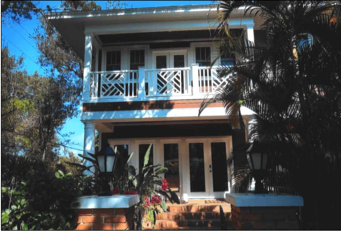
Figure 7: Rear elevation, showing new addition
