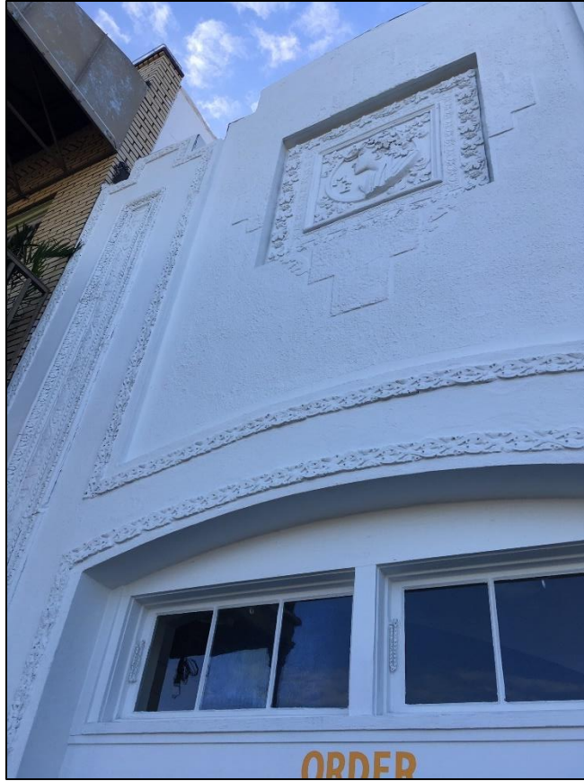
Figure 3: Detail of stucco/plaster repair
