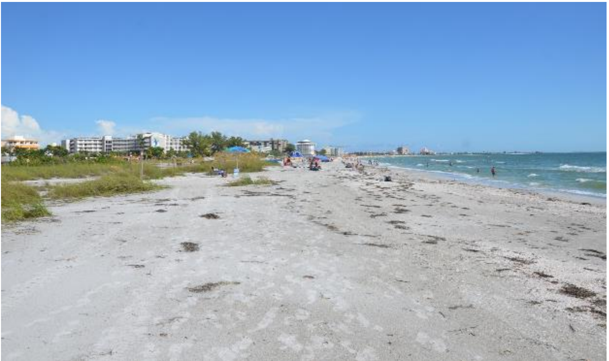
Figure 47. The T-groin #5 which was partially exposed before the storm became completely buried by “back beach overwash”, also notice the partial burial of the sea oaks due to the overwash.
