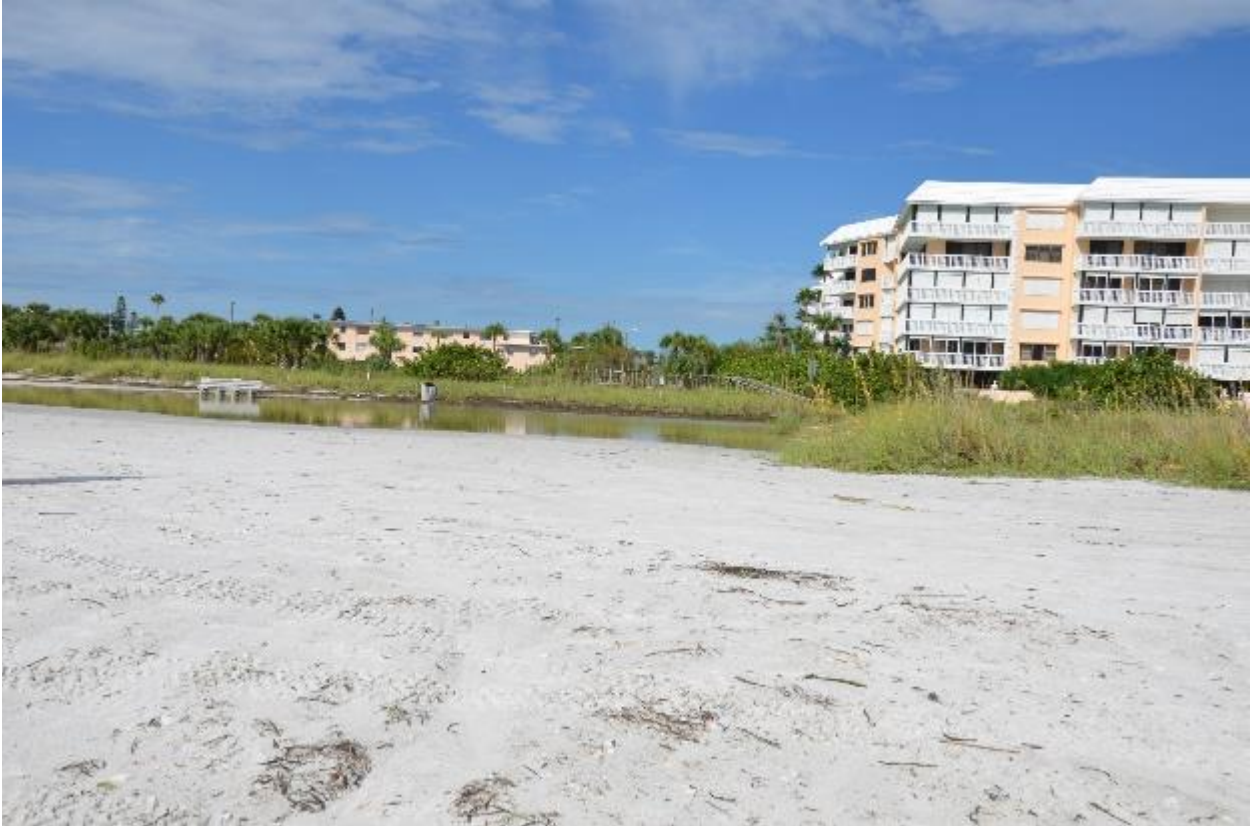
Figure 48. Flooding and ponding at the lower portion of wide back beach.
