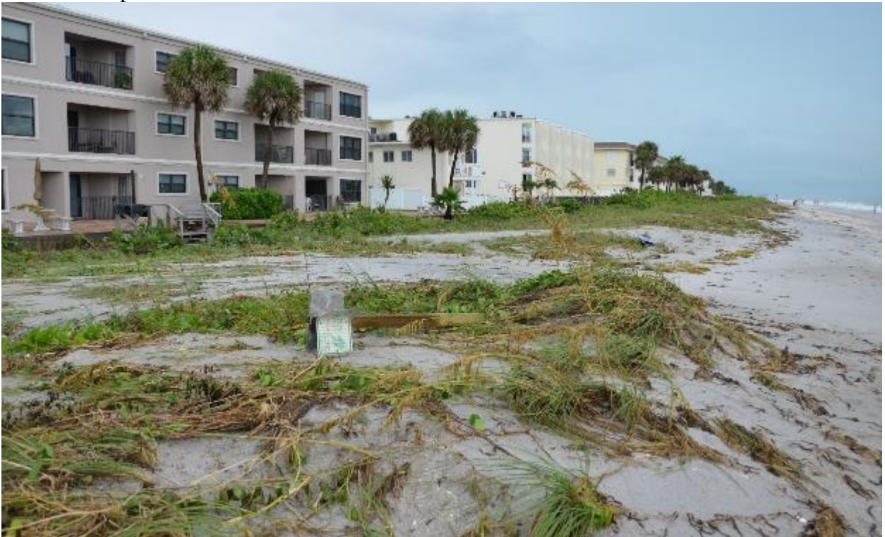
Figure 12. The low dune was overtopped by the storm water, resulting in overwash deposit in the dune field and many fell-down signs.
