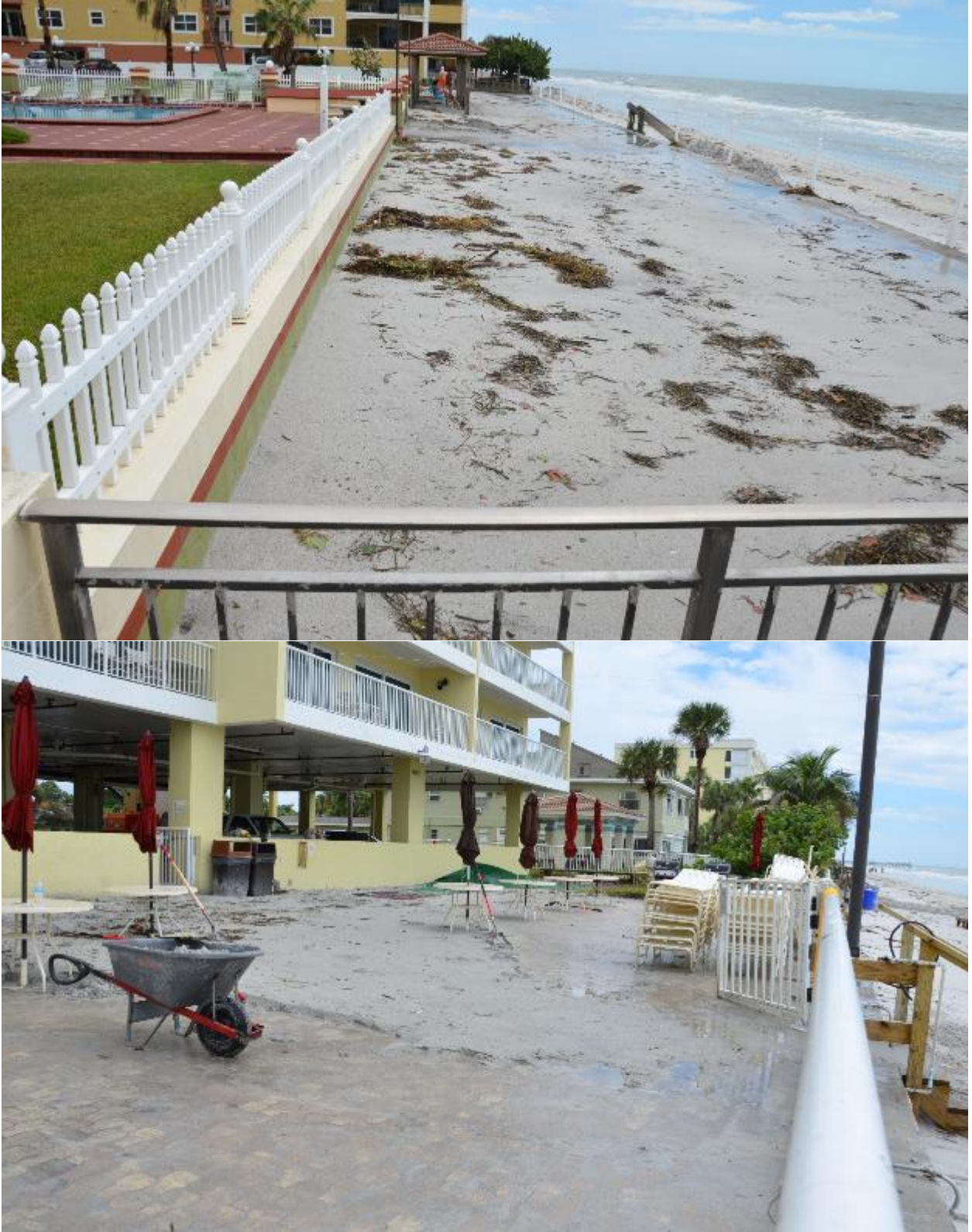
Figure 27. Sand washed onto the decks of beach front properties.
