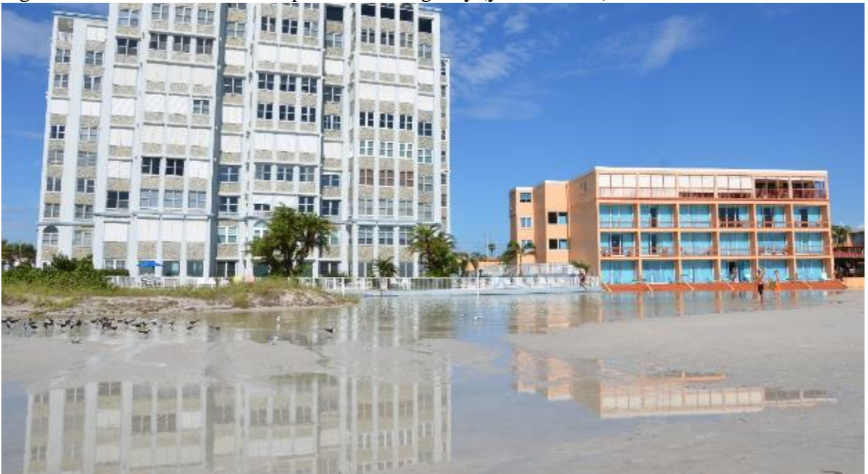
Figure 50. Flooding of the lower portion of the wide back beach in the middle Long Key.
