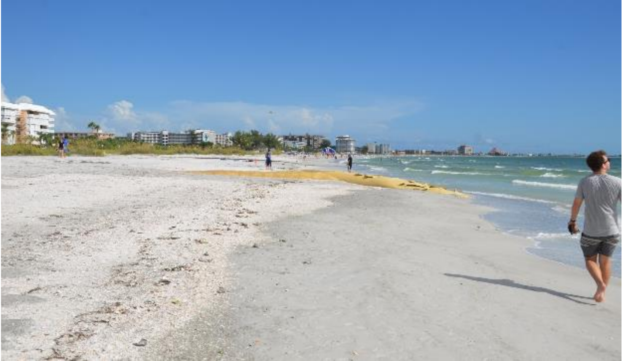
Figure 46. Severe beach erosion exposed T-groin #4, which was completely buried before the storm.
