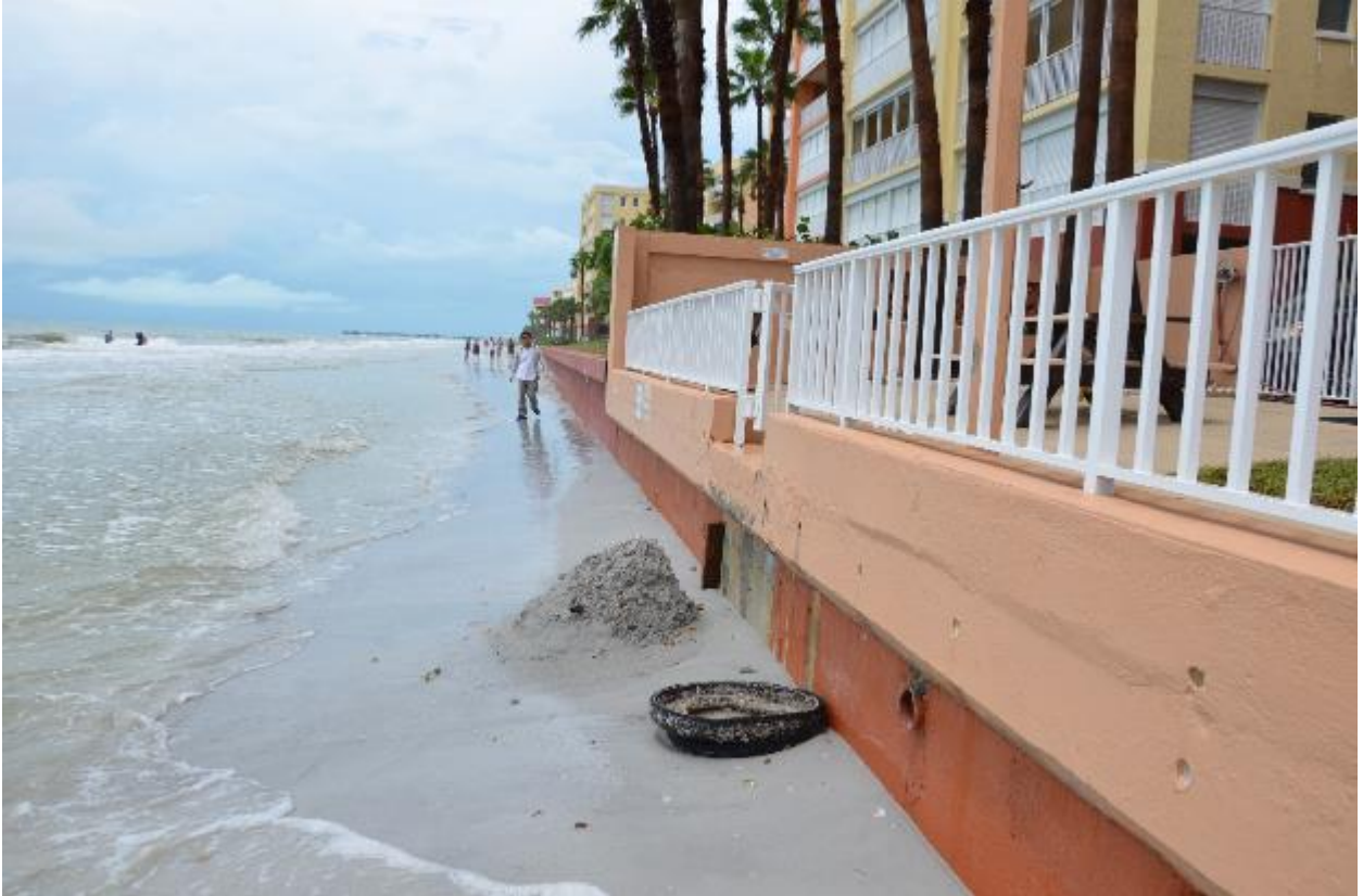
Figure 28. Severe scour along a stretch of seawall. The storm had overtopped the wall and deposited sand landward.
