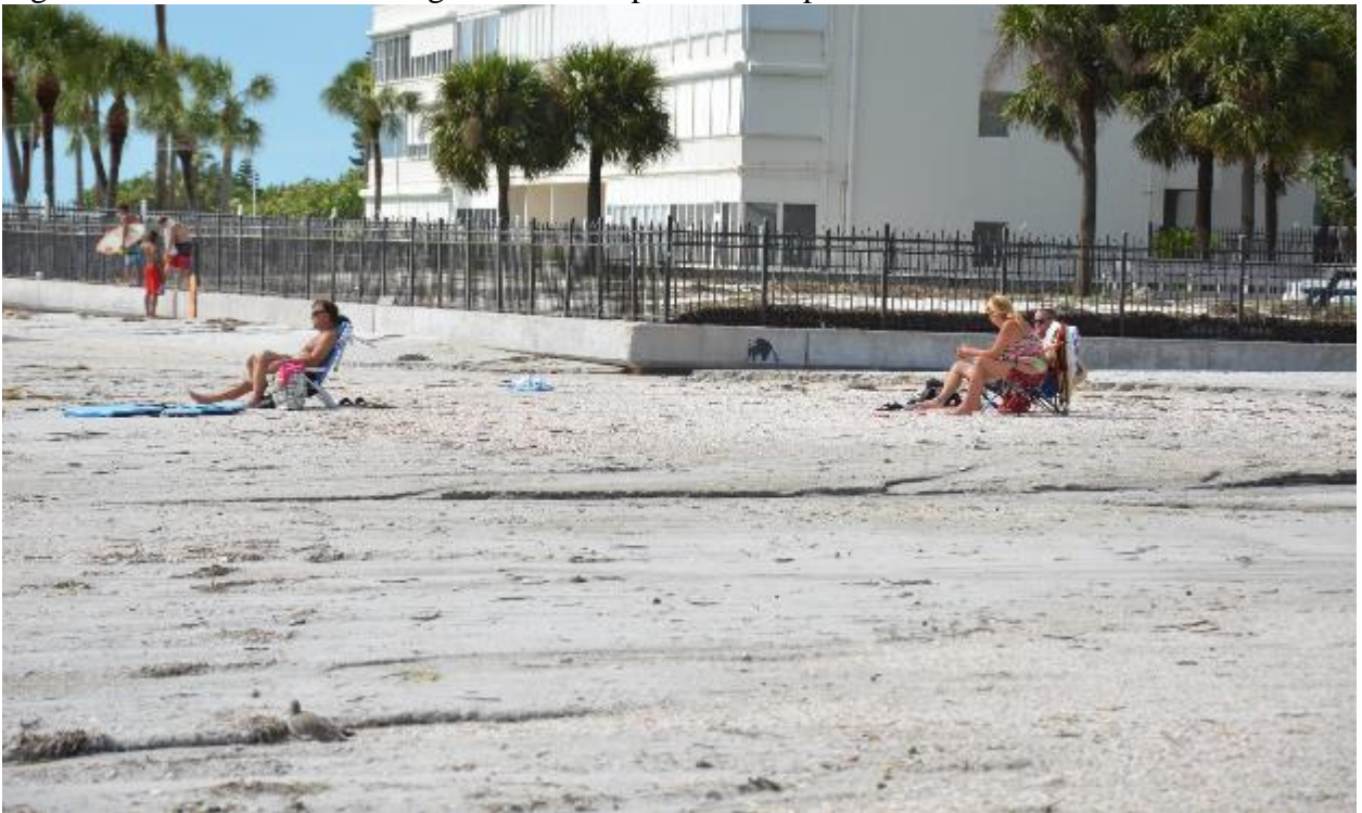
Figure 45. Large amount of sand was washed over the seawall.
