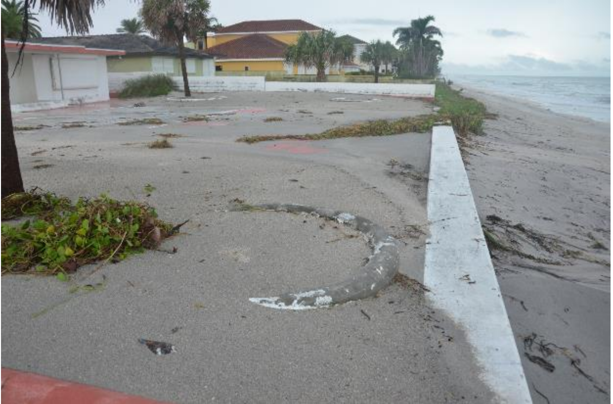
Figure 14. Sand was washed over the seawall. The narrow pre-storm beach and dune were almost completely eroded.
