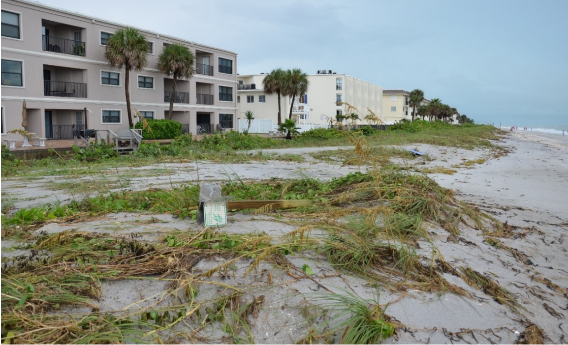
Figure 11-1: Storm overwash deposits in the dune field, landward of the seawall (Photo from USF)
