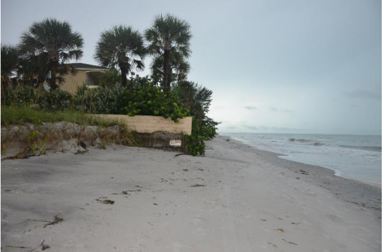
Figure 16. Erosion at a section (a neighborhood park) without seawall.
