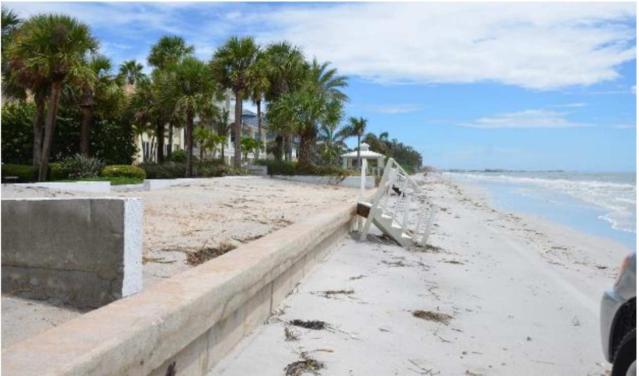
Figure 28. Severe scour along a stretch of seawall. The storm had overtopped the wall and deposited sand landward.
