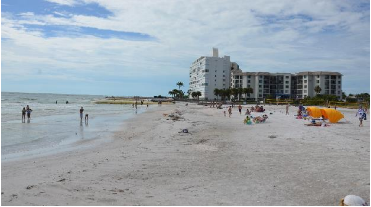
Figure 44. Beach erosion along the northern portion of Upham Beach.
