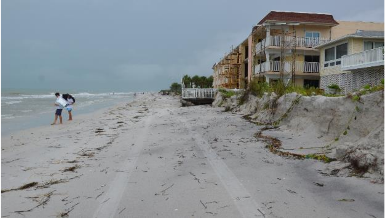
Figure 21. Severe beach and dune erosion at R84.
