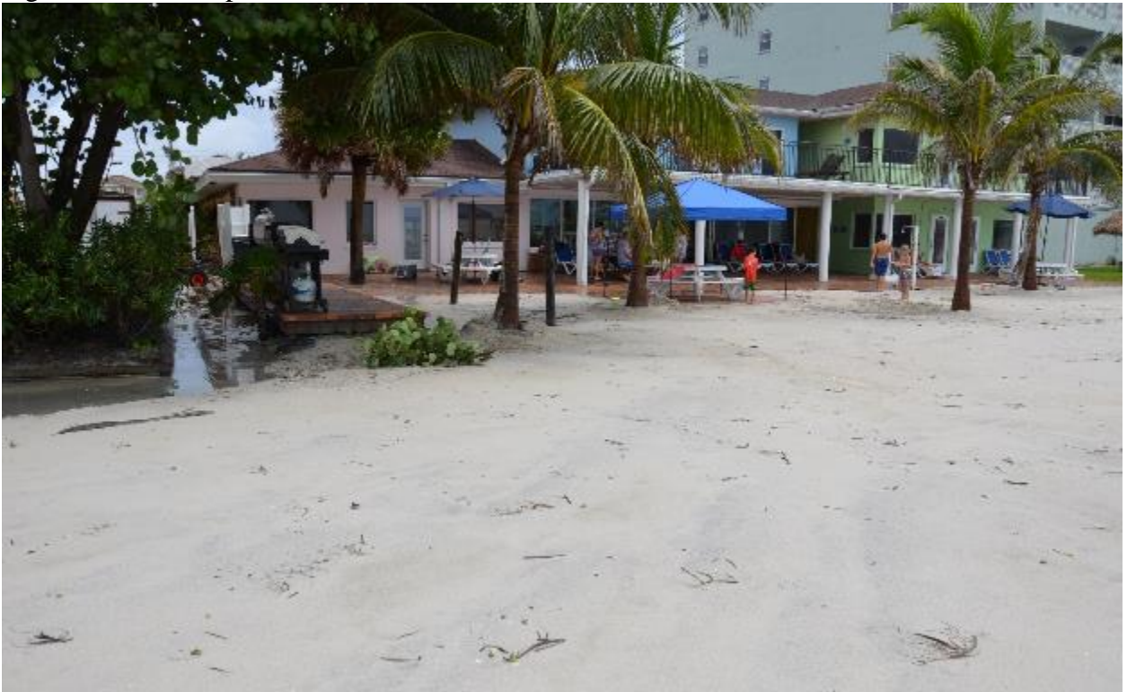
Figure 24. Sand washed over seawall along stretches without dunes.
