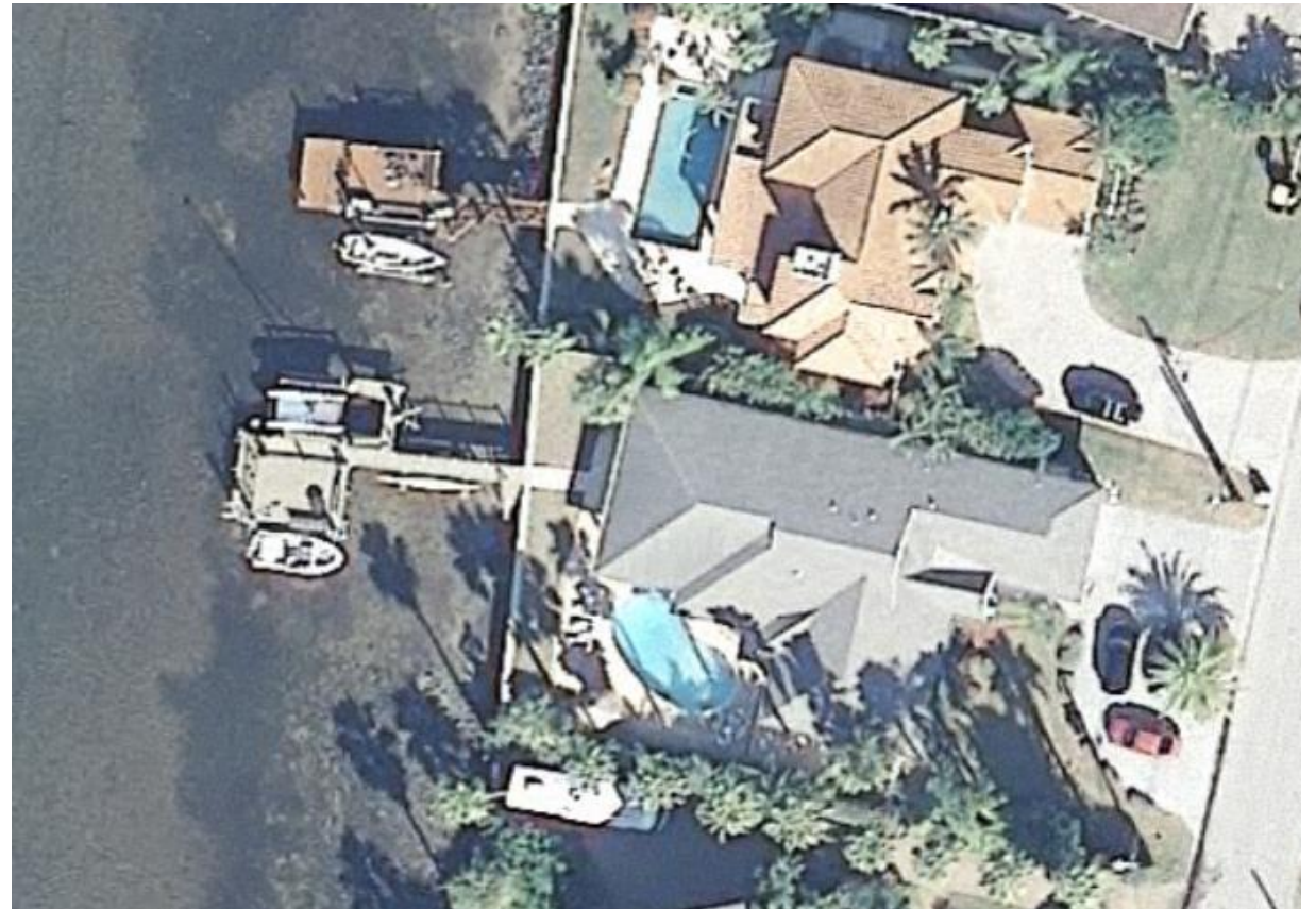
2008 – majority of stub-out removed
