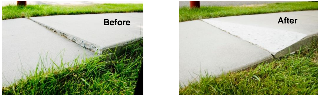
Section 3, Figure 1: Precision Sidewalk Safety Work Example
