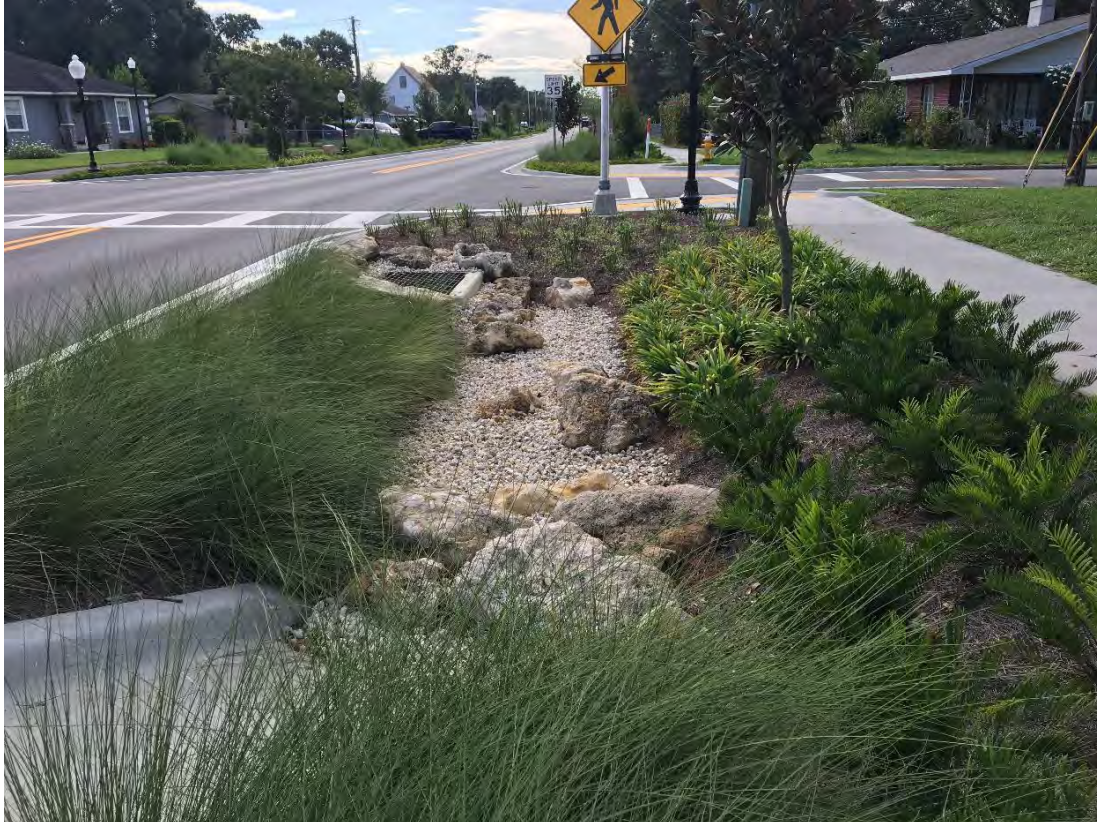
PK Avenue bioswale – Auburndale, FL
