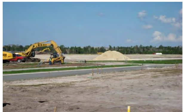
Avoid complete site clearing
