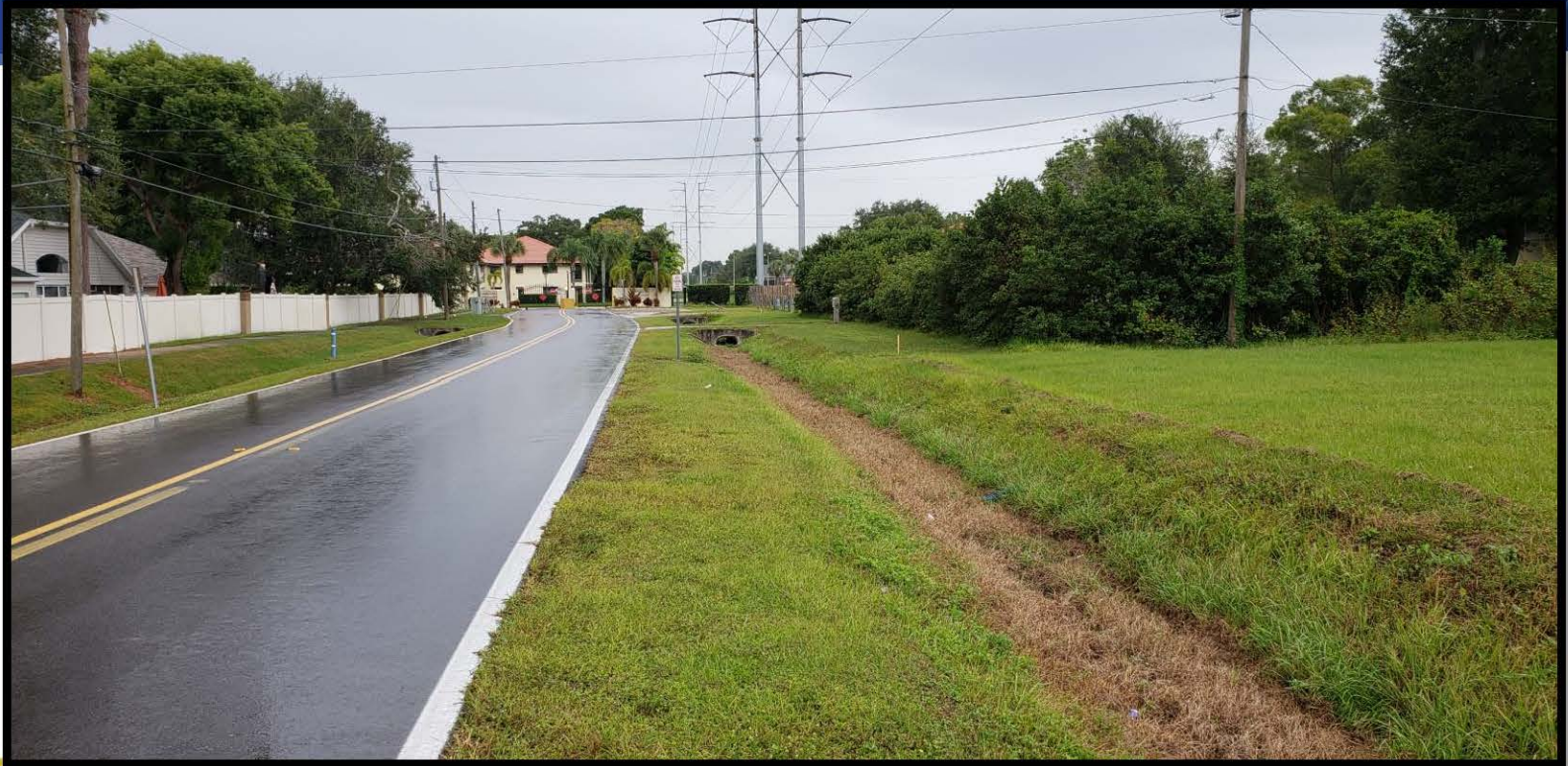
Looking north along Summerdale Dr
