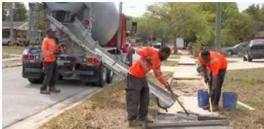
Public Works employees pouring cement for new sidewalks
