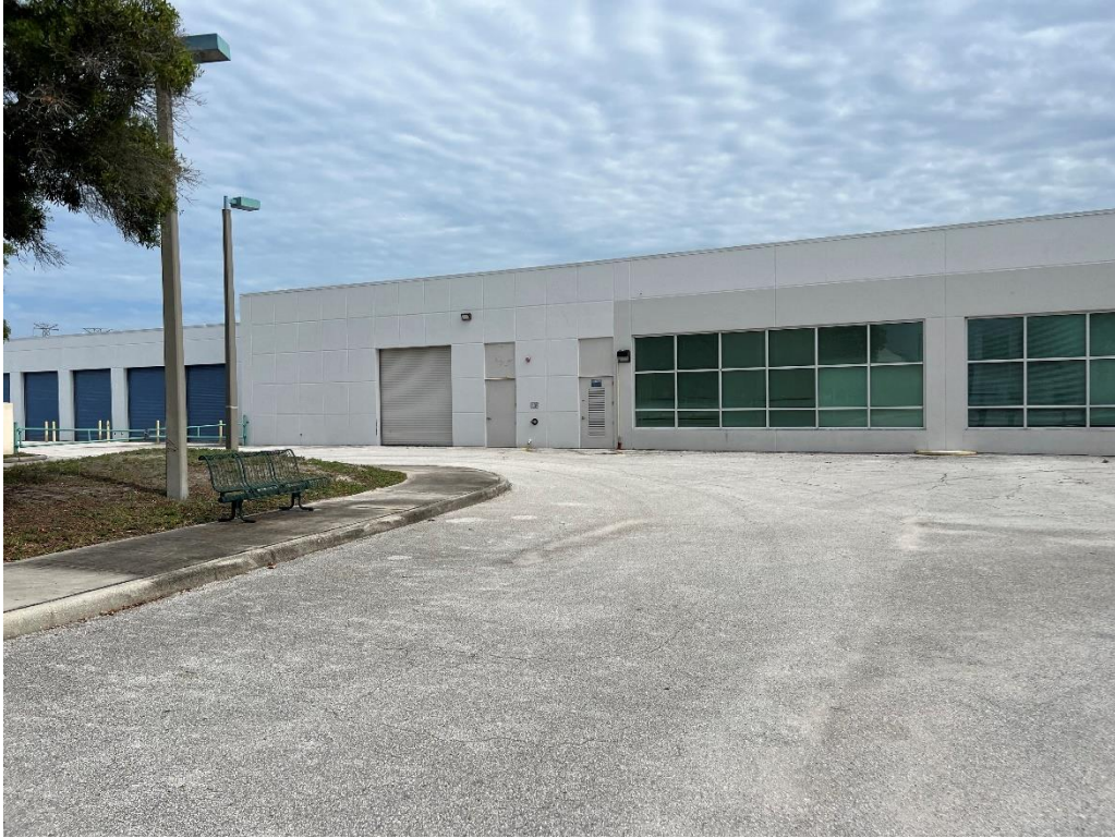
SUBJECT EXTERIOR (BUILDING 2)
