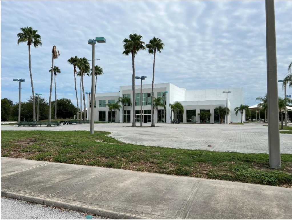
SUBJECT EXTERIOR (BUILDING 1)
