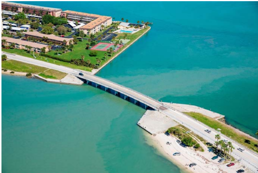
Existing Tide Relief Bridge
