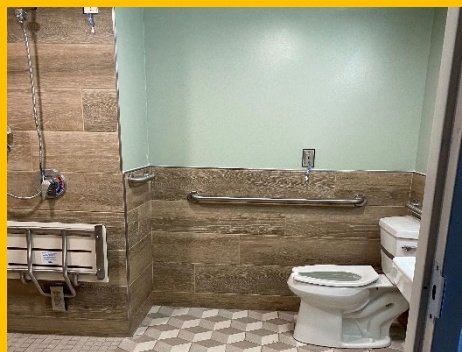
PARC Bert Muller Facility Improvements - Bathroom Renovations Phase 1
