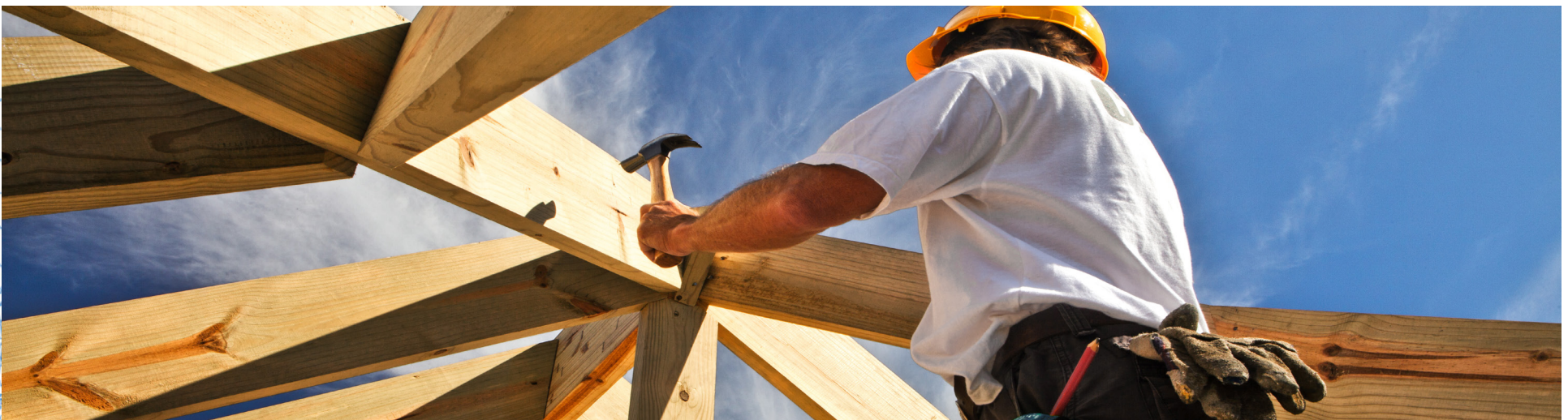
Rofer at a construction site
