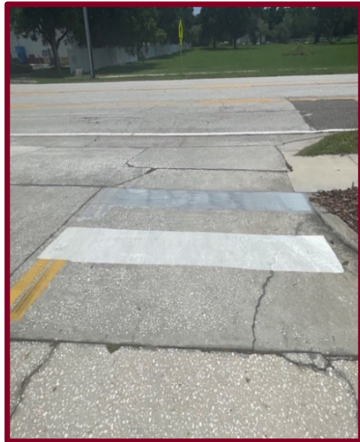
Figure 2 - Stop bar setback (original stop bar covered and moved further back)
