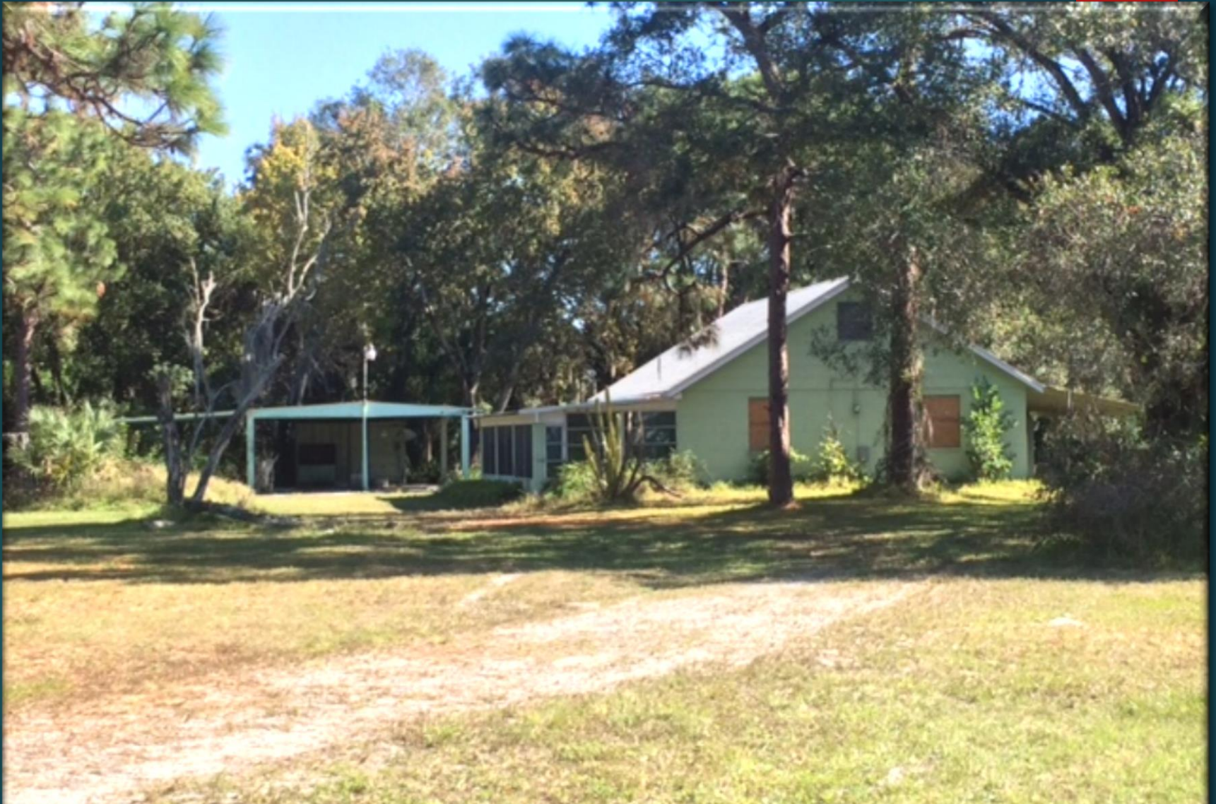
Abandoned Single Family Home
