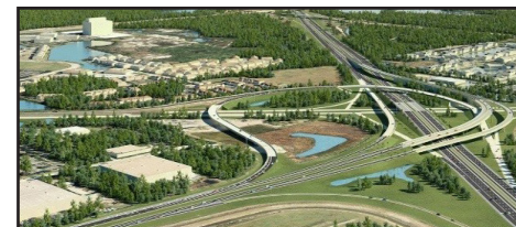
118th Avenue North Aerial View - St. Petersburg photo courtesy of Pinellas County Marketing and Communications Department
