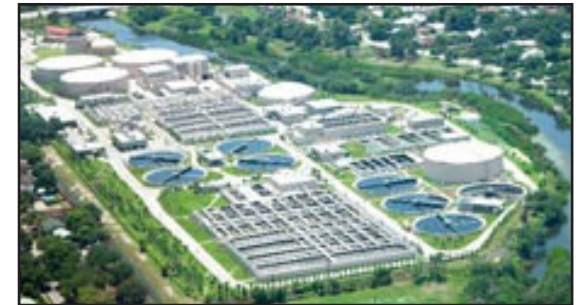
South Cross Bayou Water Reclamation Facility photo courtesy of Pinellas County Marketing and Communications Department
