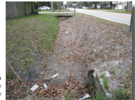
Existing Area Drainage Infrastructure
