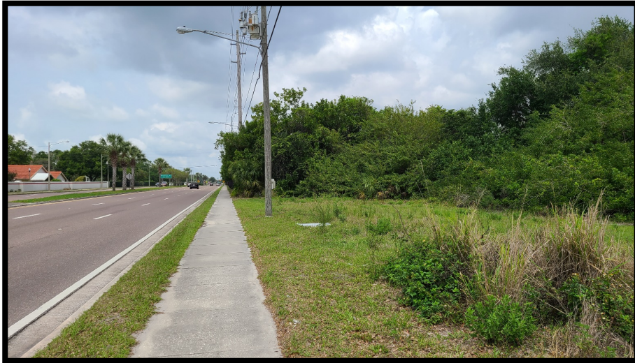
Looking north along Belcher Road
