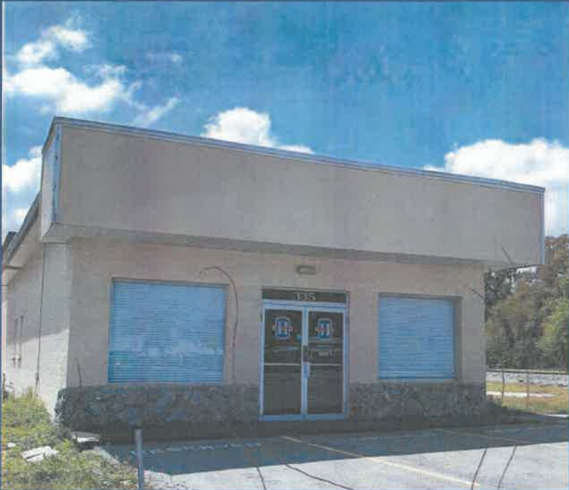
Mavrakos Office Façade Grant Before Photo
