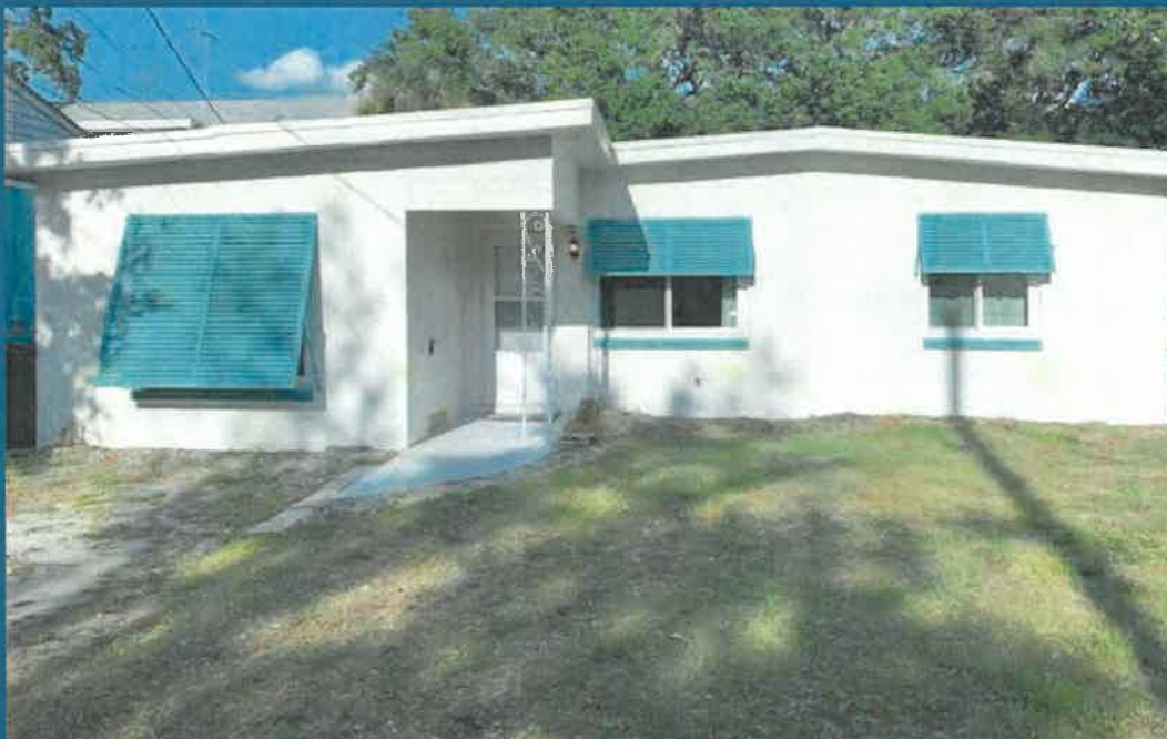
Residential Façade After Photo
