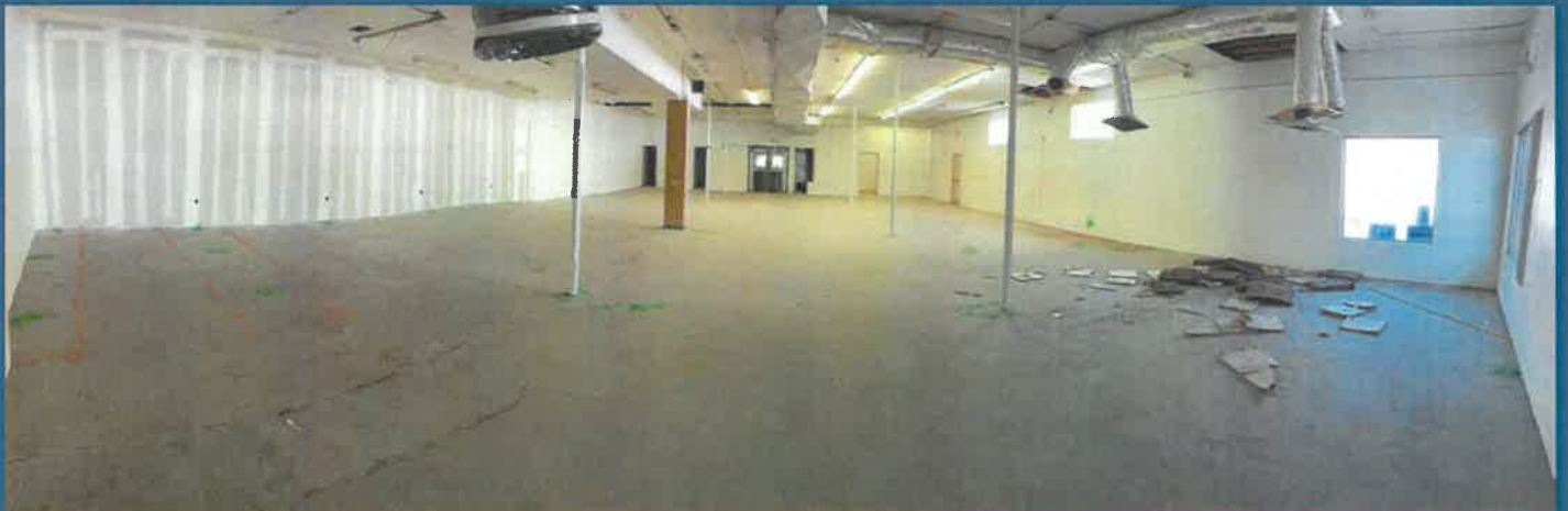
The Tides Market Interior Renovation Grant Before Photo
