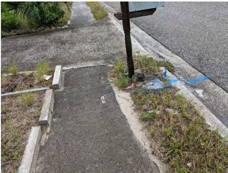
Figure 5 Inadequate Transportation Infrastructure: Sidewalk Inadequate sidewalk width, presence of utilities, lack of maintenance, sedimentation indicative of drainage issues.
