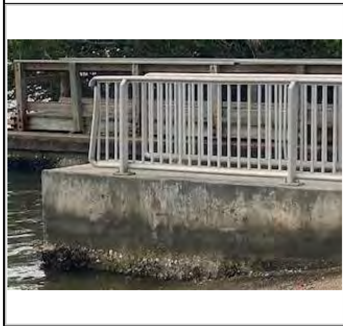
Site 1: Docks, 3 each of Gangways made of aluminum. The GPS coordinates are: 27. 8126, -82.76805; 27.48429, -82.46395; 27.48436, -82.46442., 30 FT long x 4 FT wide, Storm surge caused inundation and destabilization of the structure through increased water levels, and forceful wave action., 0% work completed.
