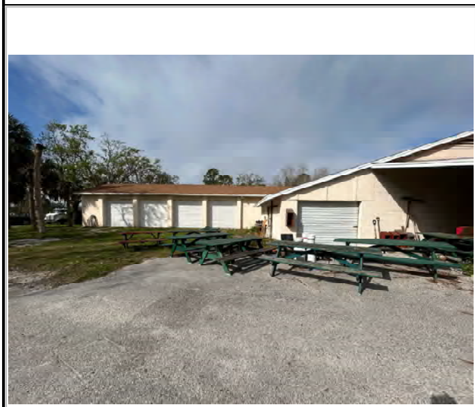
Site 2: Park Buildings, 6 each of C.H.I./3250/Ribbed Steel C.H.I. Overhead Coiling Doors, 10 FT long x 10 FT high, 3 feet of surge water pressure pushed the doors inward into the building., 100% work completed.
