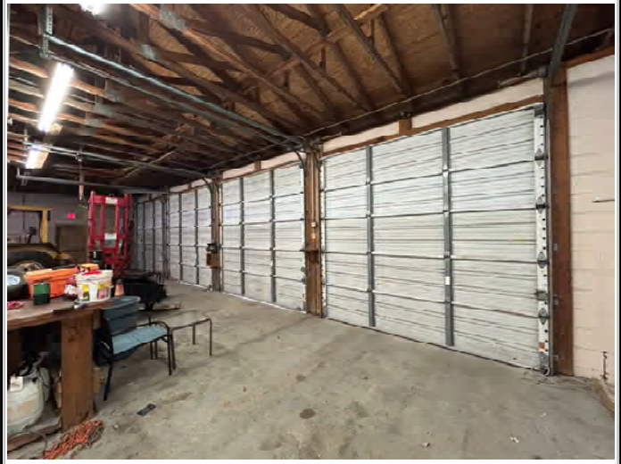
Site 2: Park Buildings, 6 each of C.H.I./3250/Ribbed Steel C.H.I. Overhead Coiling Doors, 10 FT long x 10 FT high, 3 feet of surge water pressure pushed the doors inward into the building., 100% work completed.
