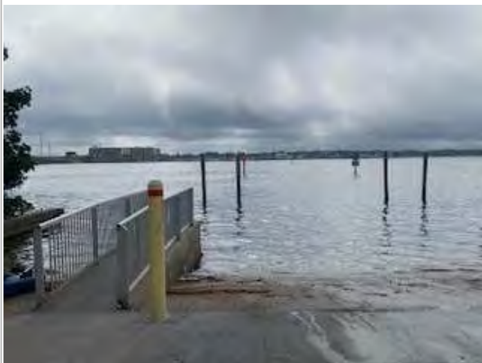
Site 1: Docks, 3 each of Gangways made of aluminum. The GPS coordinates are: 27. 8126, -82.76805; 27.48429, -82.46395; 27.48436, -82.46442., 30 FT long x 4 FT wide, Storm surge caused inundation and destabilization of the structure through increased water levels, and forceful wave action., 0% work completed.
