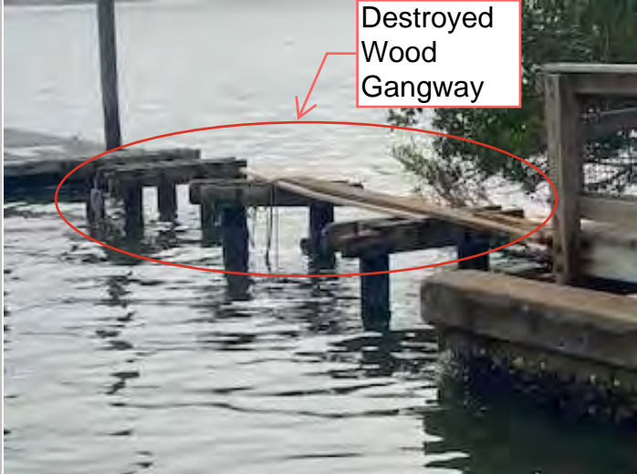
Site 1: Docks, 1 each of Wood Gangway. The GPS coordinates are: 27.81206, -82.76805; 27.48429, -82.46395; 27.48436, -82.46442., 40 FT long x 5 FT wide, Storm surge caused inundation and destabilization of the structure through increased water levels, and forceful wave action., 0% work completed.
