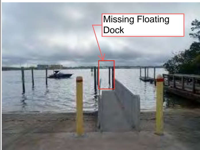
Site 1 Docks, 3 each of Missing floating docks made of wood and aluminum. The GPS coordinates are: 27.48428, -82.46421; 27.48432, -82.46424; 27.48435, -82.46404, 30 FT long x 10 FT wide, Storm surge caused inundation and destabilization of the structure through increased water levels, and forceful wave action., 0% work completed.
