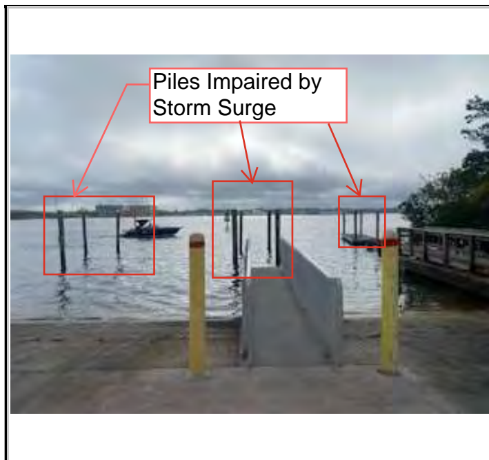
Site 1 Docks, 16 each of Piles, made of wood and are 13 feet high. The GPS coordinates are: 27.48442, -82.46675., 13 FT high, Storm surge caused inundation and destabilization of the structure through increased water levels, and forceful wave action., 0% work completed.
