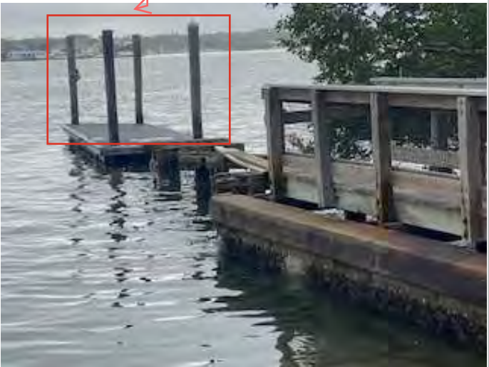
Site 1: Docks, 1 each of Wood/Aluminum Floating Dock. Wood & aluminum deck with corrugated metal filled pontoons. The GPS coordinates are 27.48423, -82.46395., 30 FT long x 10 FT wide, Storm surge caused inundation and destabilization of the structure through increased water levels, and forceful wave action., 0% work completed.
