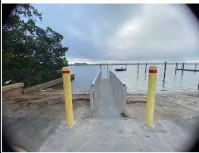
Site 1: Docks, 3 each of Gangways made of aluminum. The GPS coordinates are: 27. 8126, -82.76805; 27.48429, -82.46395; 27.48436, -82.46442., 30 FT long x 4 FT wide, Storm surge caused inundation and destabilization of the structure through increased water levels, and forceful wave action., 0% work completed.
