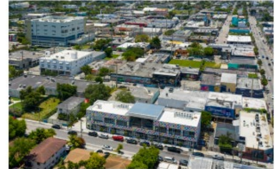
Industrial mixed-use areas maintain warehouse and light manufacturing uses, but can also include live/work units and artisan co-working spaces/studios. Murals can create a sense of place and make the area more attractive to activity.
