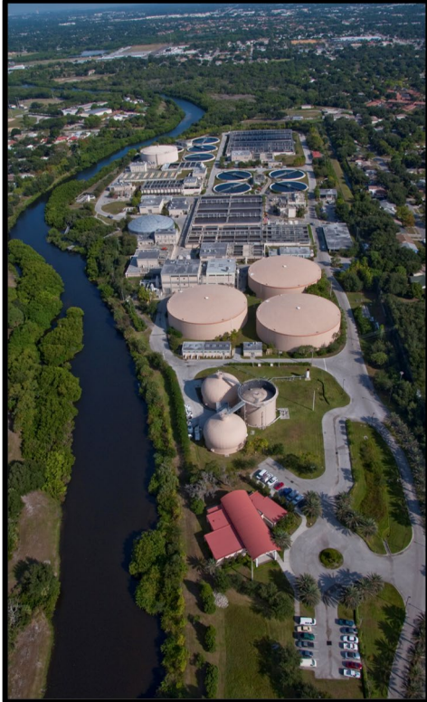
South Cross Bayou Advanced Water Reclamation Facility
