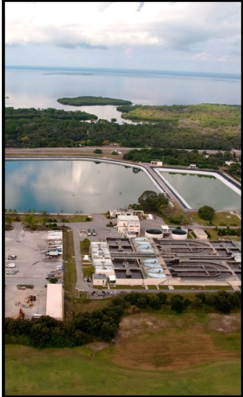
W.E. Dunn Water Reclamation Facility
