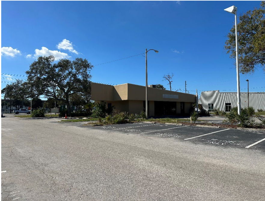
Photo 1: Taken from the northeast portion of the property.
