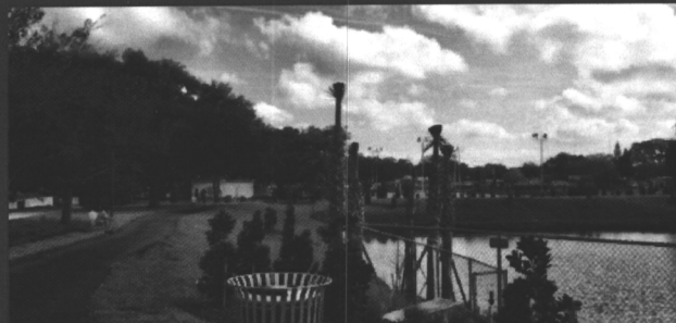
New Landscaping & Hardscaping improvements for stormwater ponds
