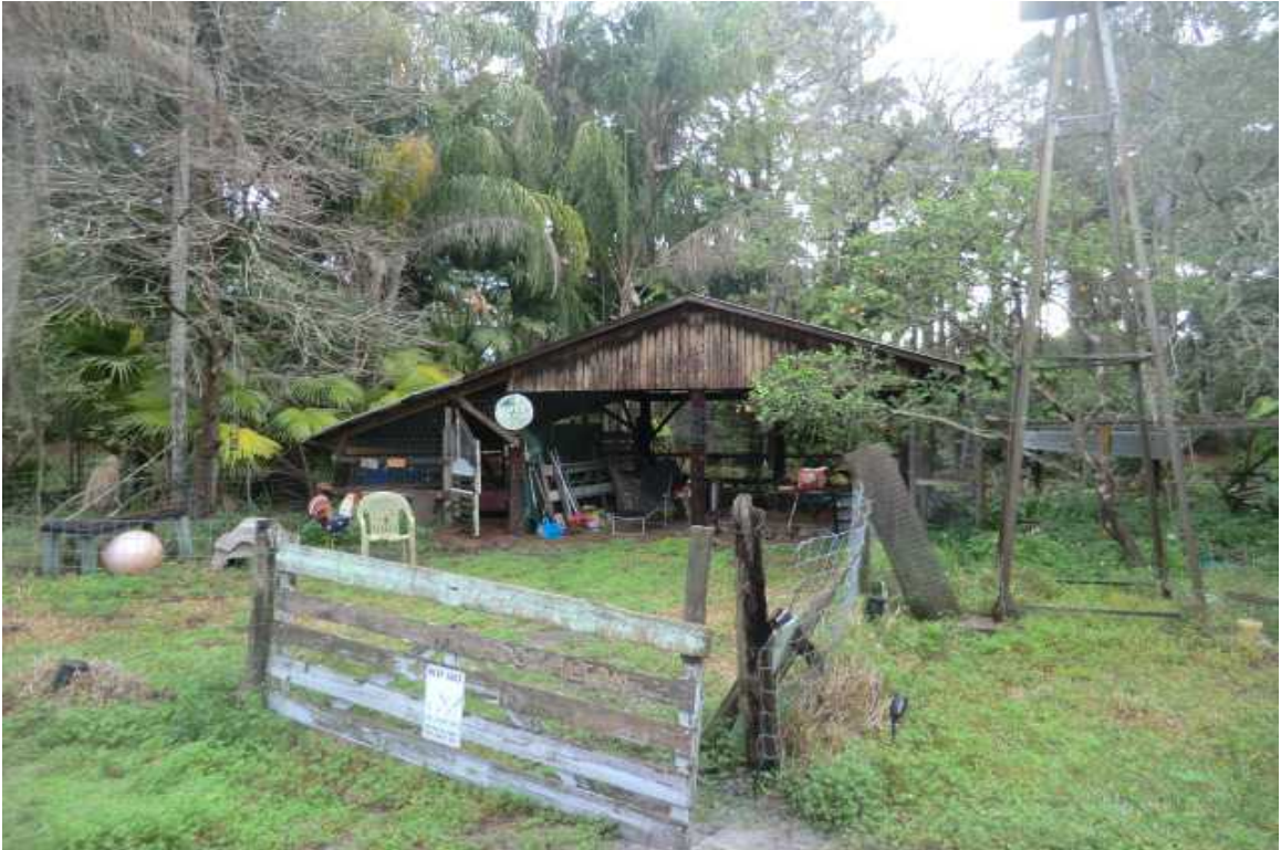
BARN ON PROPERTY
