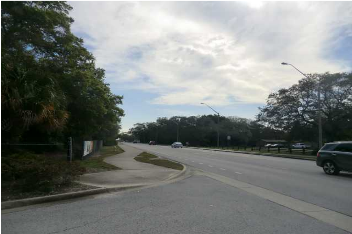
WALSINGHAM ROAD - FACING EAST
