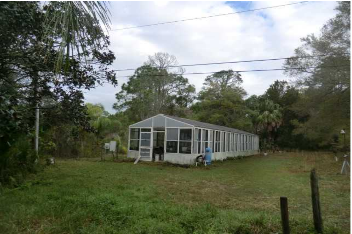
GREENHOUSE ON PROPERTY
