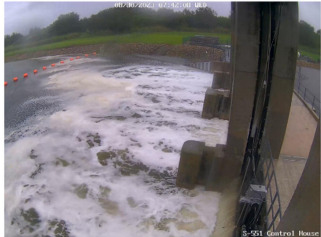
Tidal storm surge overtopping the S-551 structure during Hurricane Idalia in 2023
