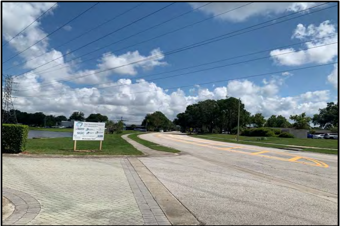
VIEW NORTH ON ICOT BLOULEVARD FROM SUBJECT PROPERTY
