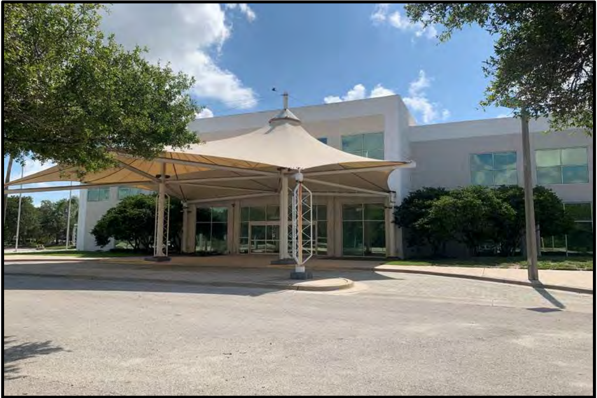
BUILDING A; WEST FACADE
