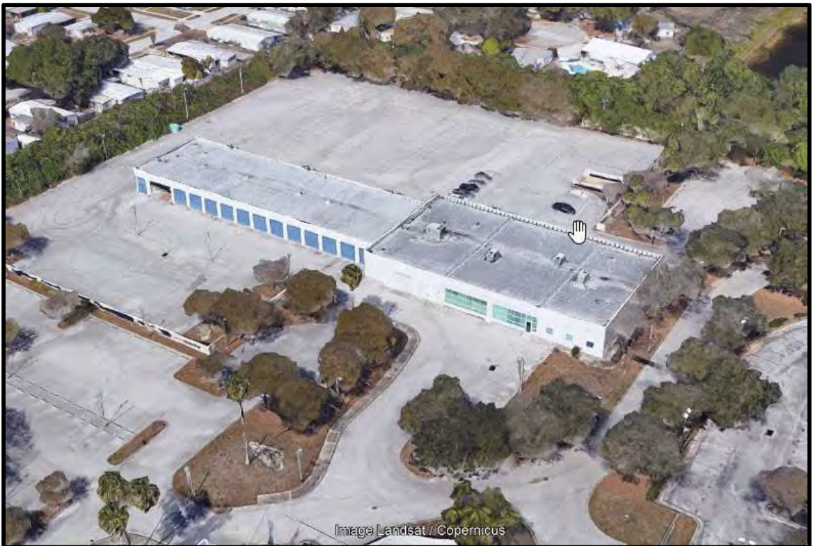
AERIAL VIEW OF BUILDING B FROM SOUTHEAST
