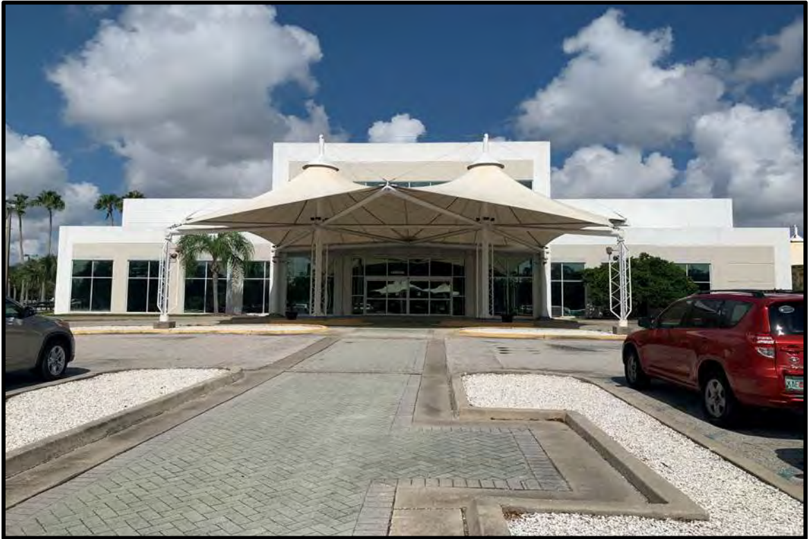
BUILDING A; EAST FACADE
