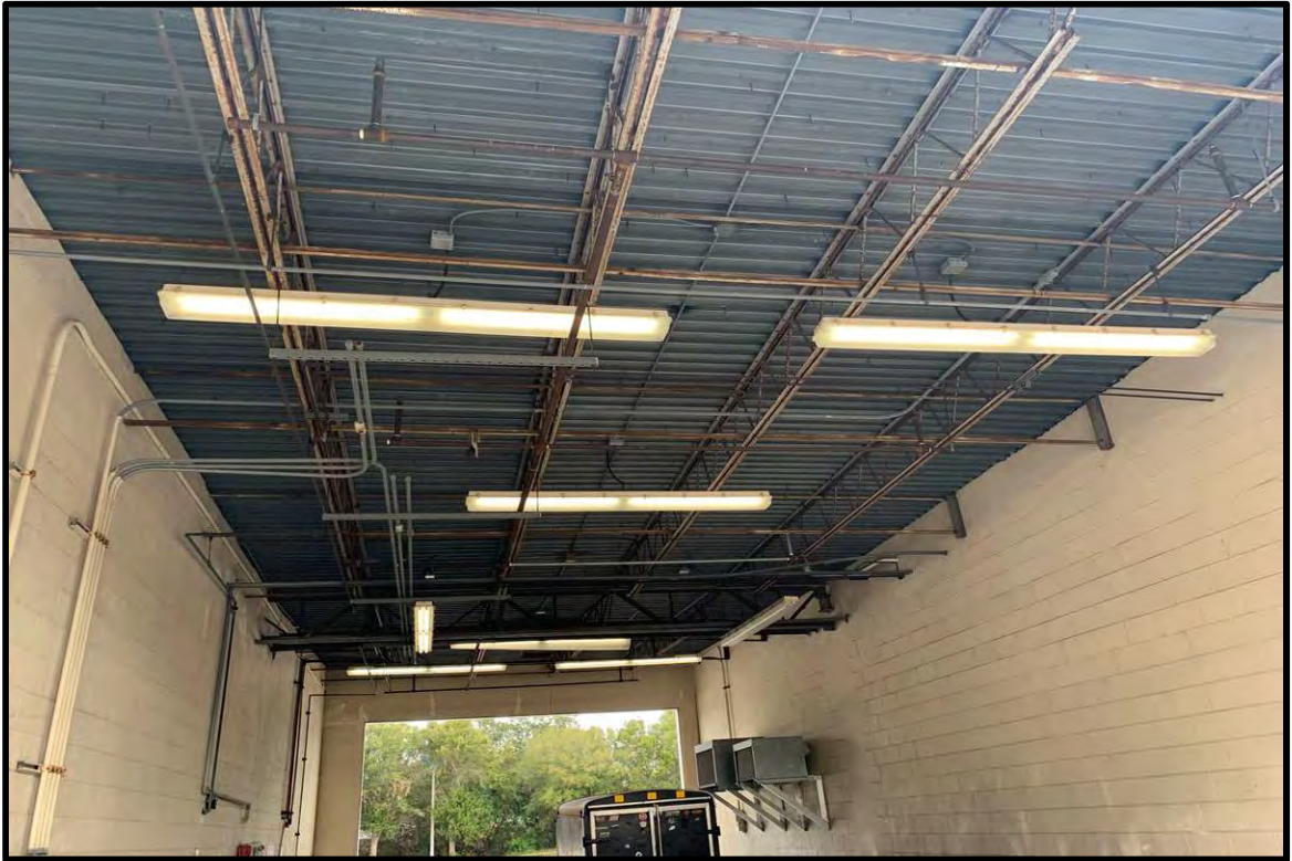
TYPICAL SERVICE BAY INTERIOR IN WEST SECTION OF BUILDING B
