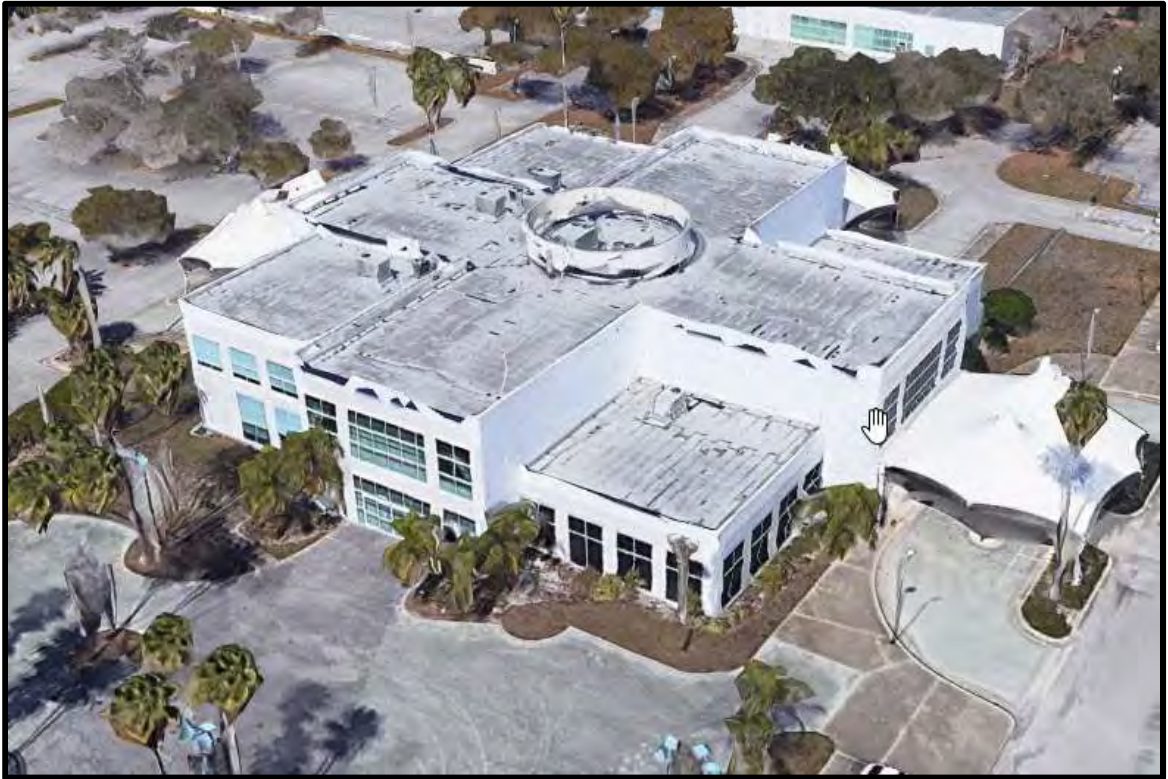
AERIAL VIEW OF BUILDING A FROM SOUTHEAST
