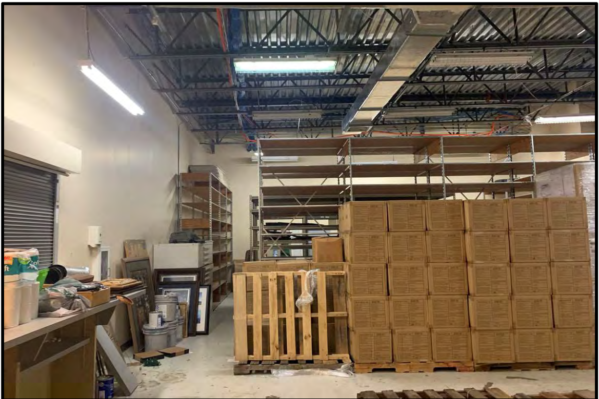
BUILDING B; TYPICAL WAREHOUSE FINISHES
