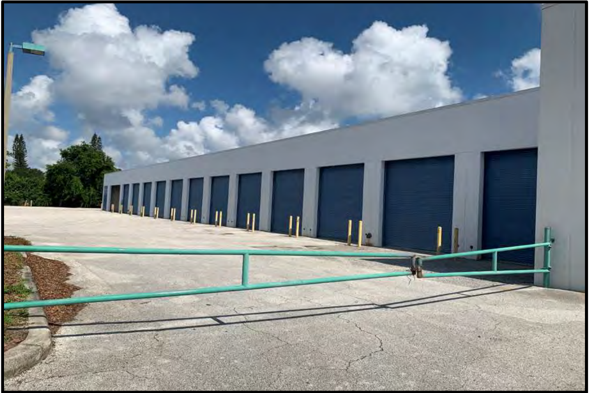
BUILDING B; WEST SECTION OF SERVICE BAYS
