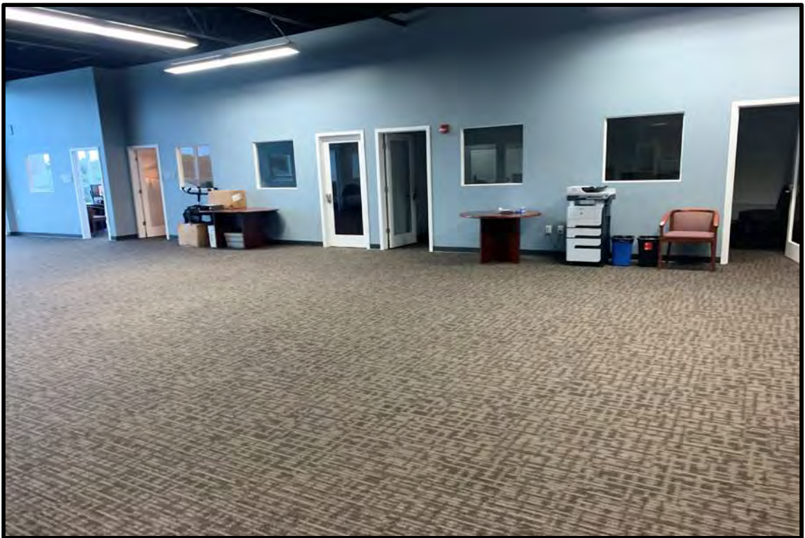
BUILDING A; OVERLY BROAD CORRIDORS ON 2 ND FLOOR
