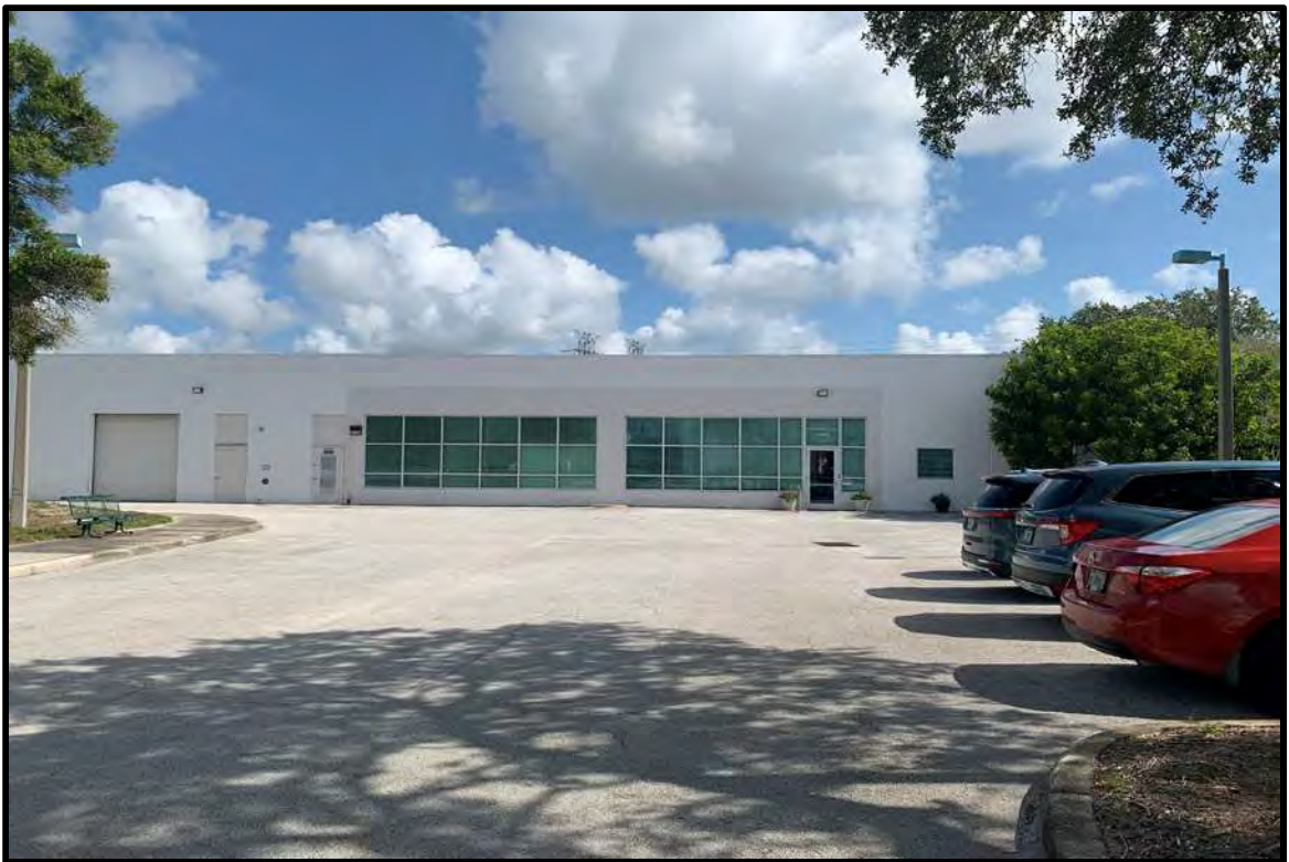
BUILDING B; EAST SECTION FLEX SPACE
