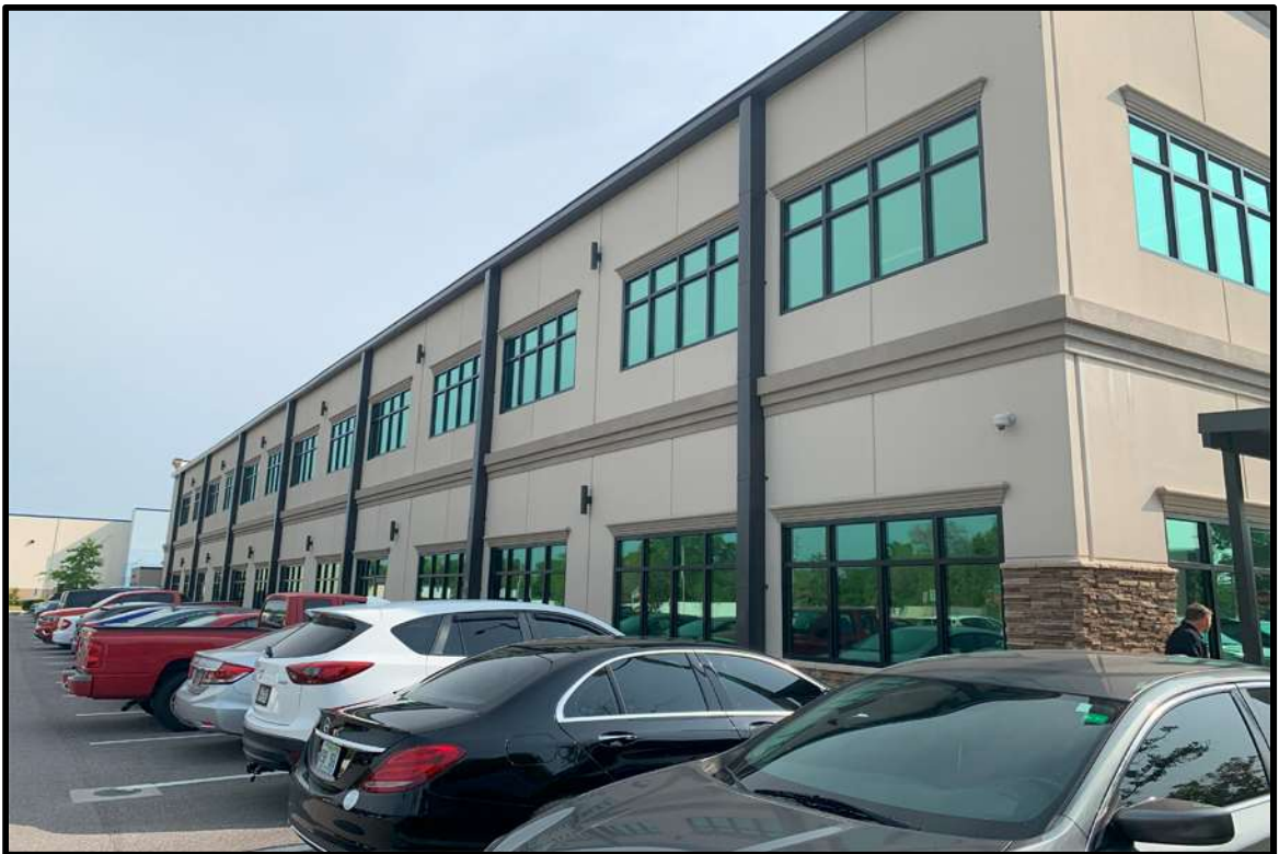
REAR VIEW FROM SOUTHWEST
