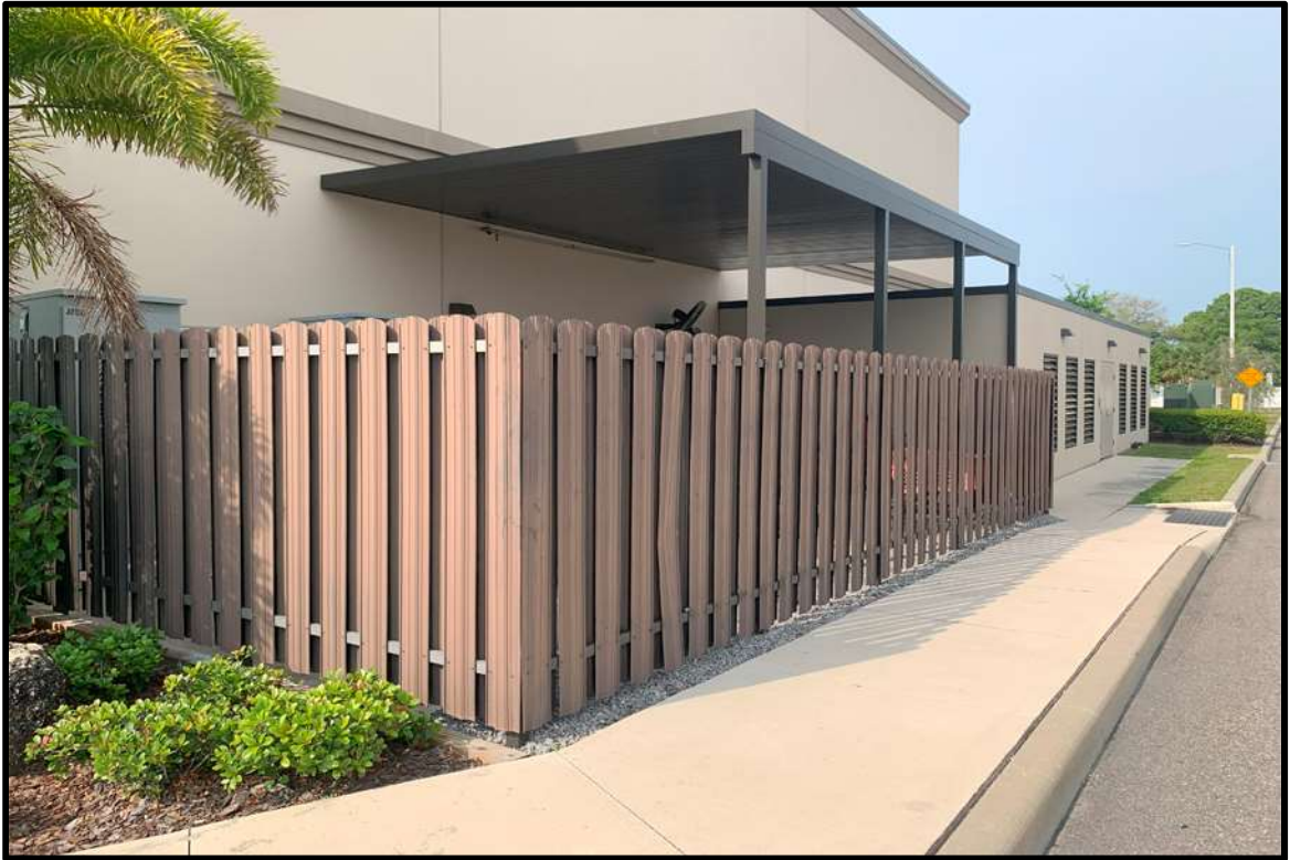
STAFF BREAK AREA WITH CANOPY AT NORTHEAST CORNER
