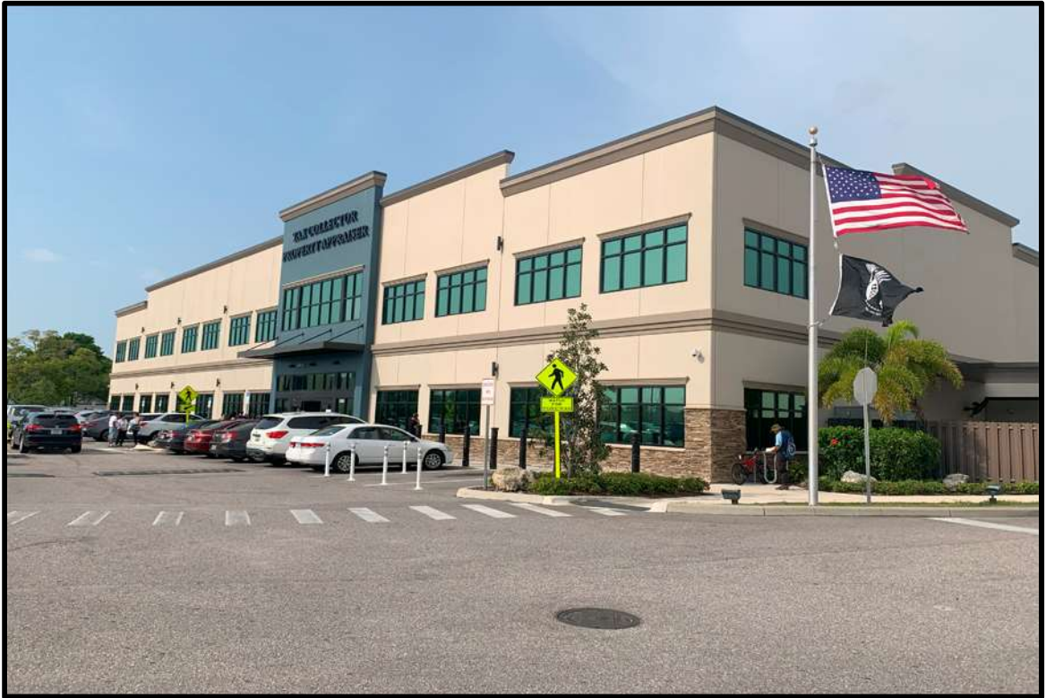
BUILDING DETAIL VIEW FROM NORTHEAST
