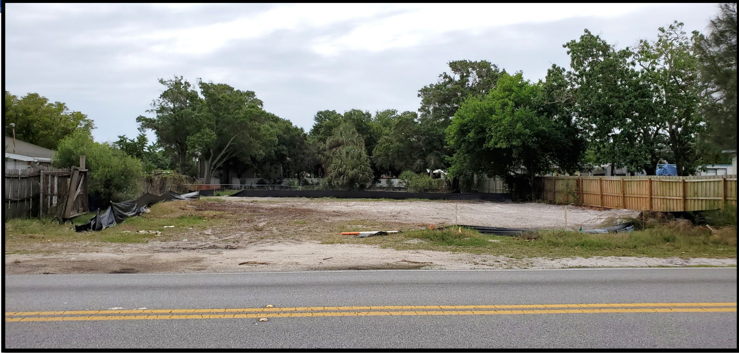
Looking east at subject property from 28 th Street North
