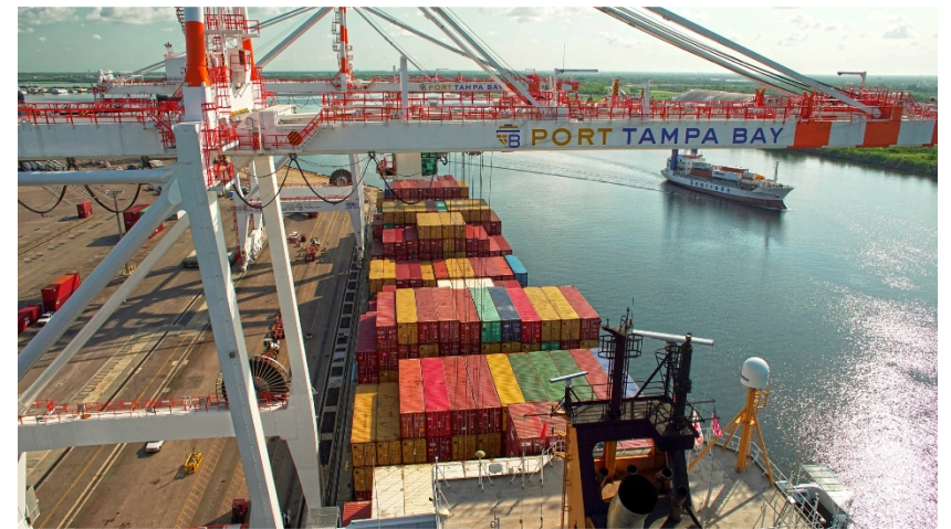
Post-Panamax container cranes
