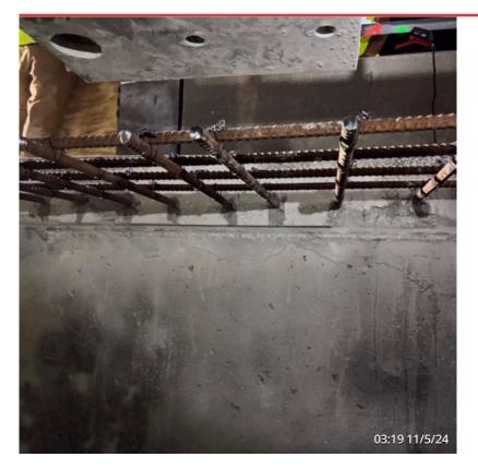
ISSUE 20 Storm Damage Repair Rebar installed, tied and epoxied
