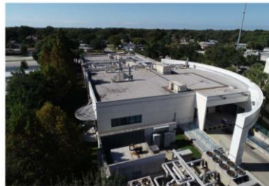
Photograph 3 - Partial Left Elevation
