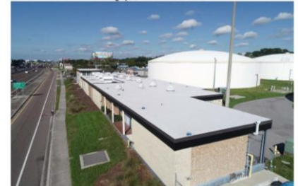
Photograph 2 - Partial Front Elevation
