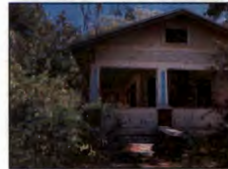
Figure 19: Deterioration of Site Conditions within the CRD Source: Kimley-Horn
