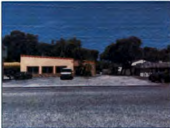
Figure 14: Parking Lot with a Large Driveway Width in the CRD Source: Kimley-Horn
