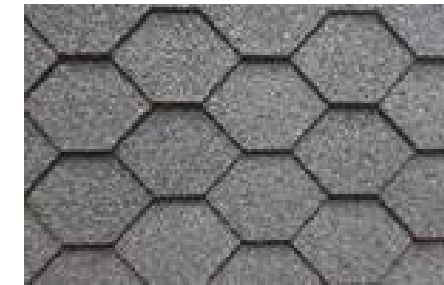
Asphalt shingle, diamond or hexagonal
