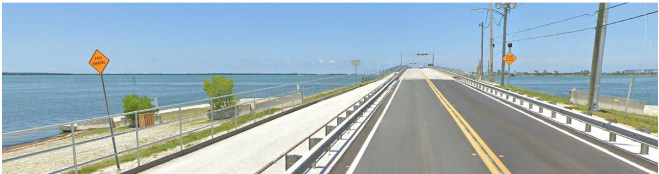
Figure 5. Bridge Street View
