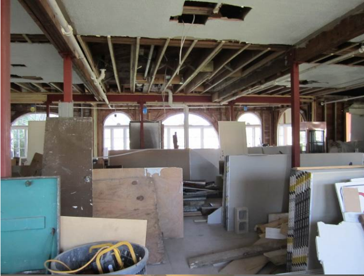
Photos 8, 9: Before/after repairs to dining room/kitchen area.
