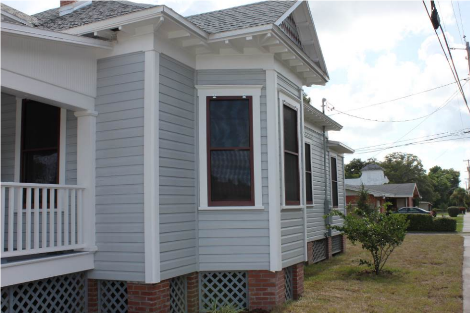
Photo 1e: Post-rehabilitation side elevation and bay window.
