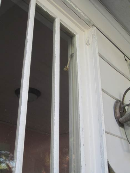
Photo 2a: Inoperable window. Photo 2b: Deteriorated window structure.
