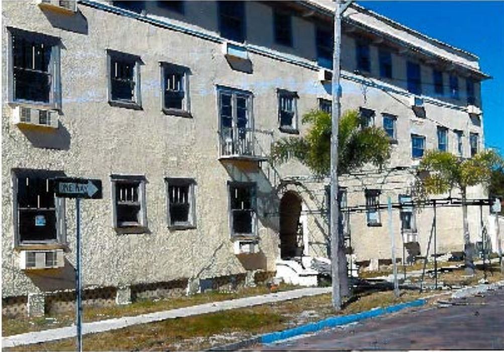
Photo 1: Before exterior cladding repairs.
