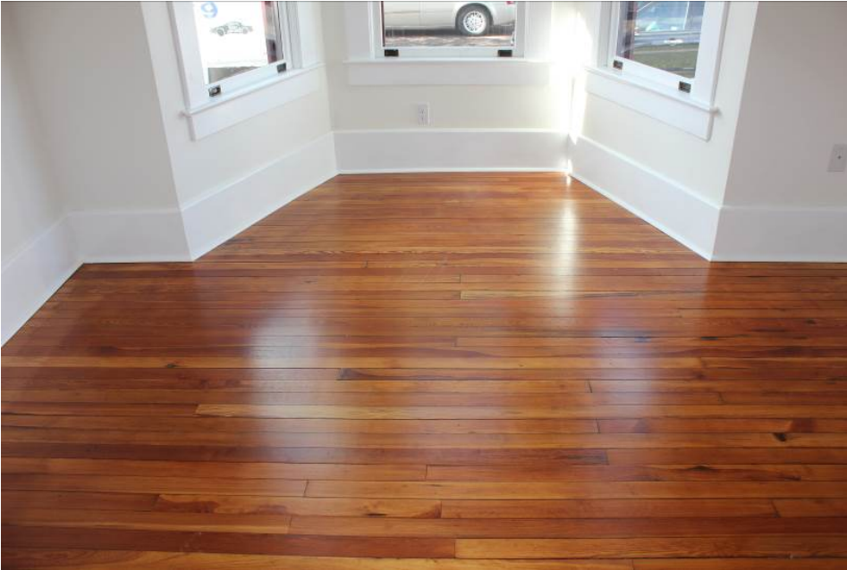
Photo 2b: Post-rehabilitation wood flooring (typ.).
