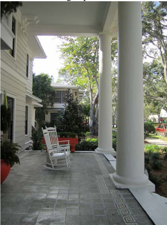
Photo 5c: Repaired historic porch tile.
