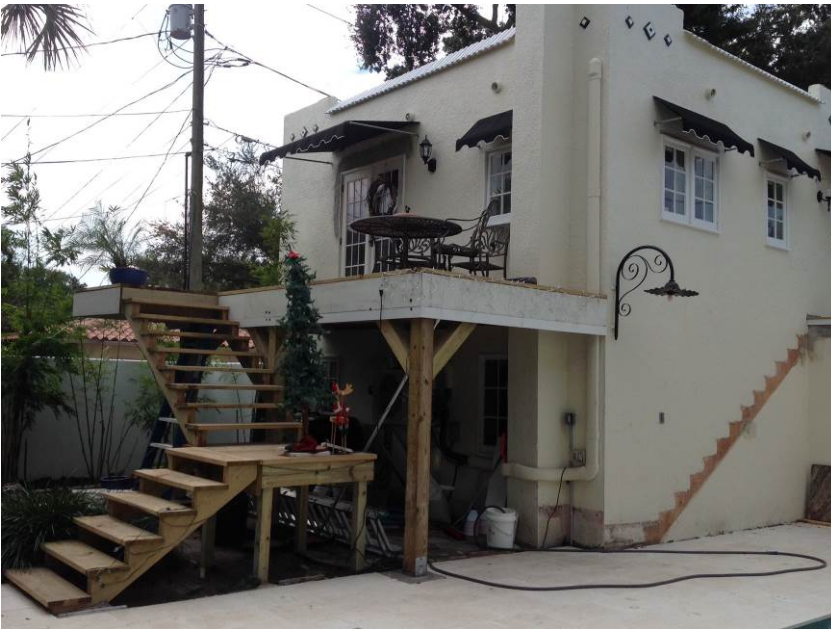
Photo 4b. Post-rehabilitation garage apartment with new deck and stair system (partial).
