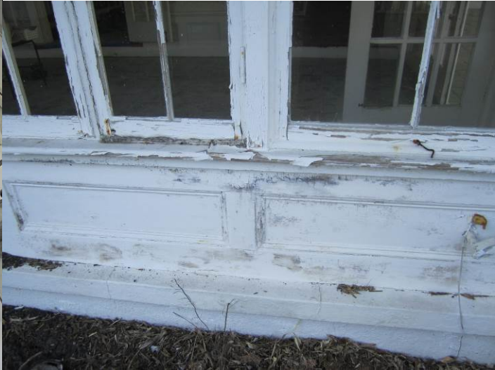
Photo 2a: Inoperable window. Photo 2b: Deteriorated window structure.
