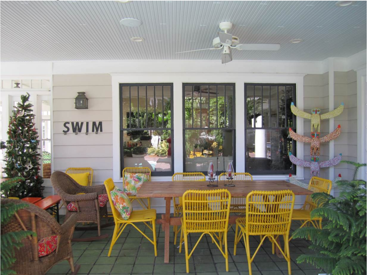
Photo 2c: Typical windows restored.
