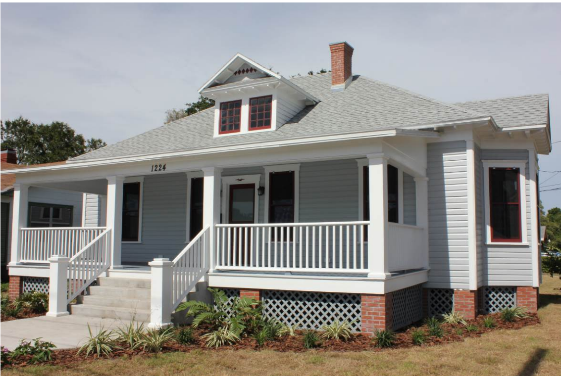
Photo 1d: Post-rehabilitation frontal elevation with open porch restoration.
