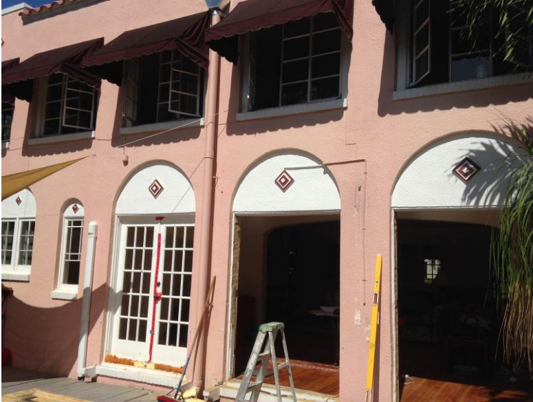
Photo 1a. Pre-rehabilitation window and door sets at rear elevation.
