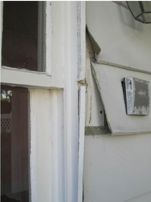
Photo 4c: Incompatible alum. cladding.
