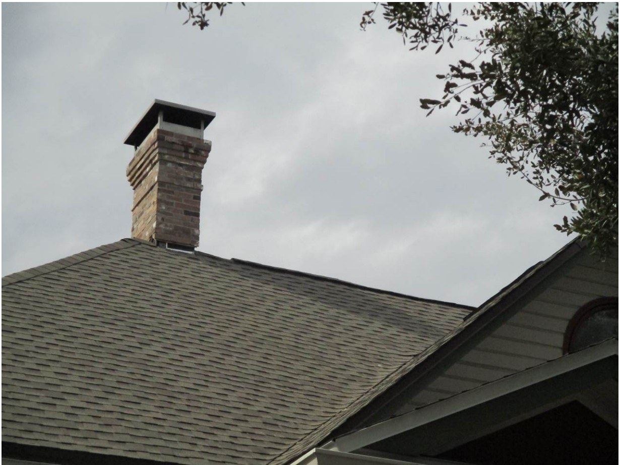
Photo 1: Repaired roof and reconstructed chimney (typ.).
