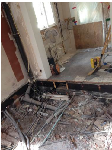
Photo 6b. Extent of damage under repair (typ.).
