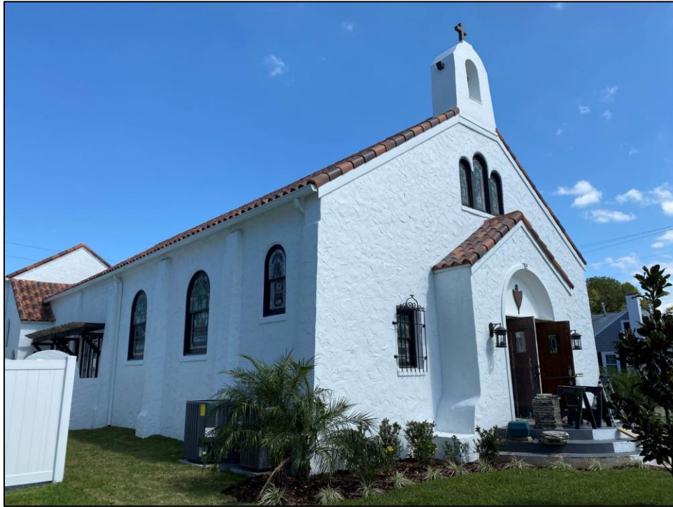
Figure 11: Façade and west elevation
