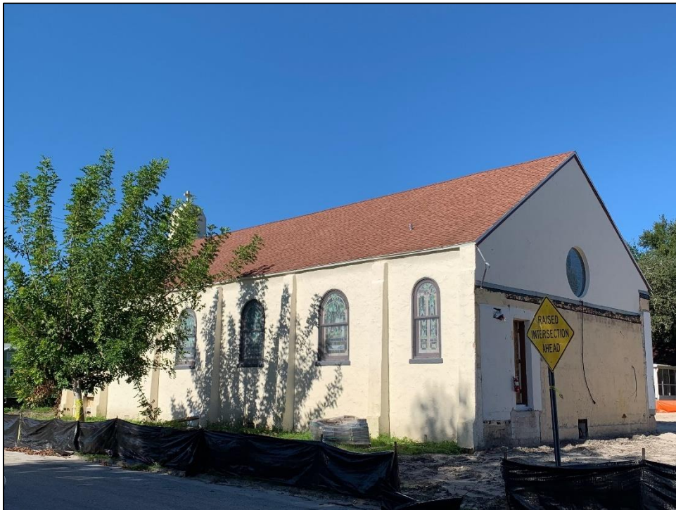
Figure 5: East (side) and north (rear) elevations of subject property following removal of non-historic additions, prior to rehabilitation
