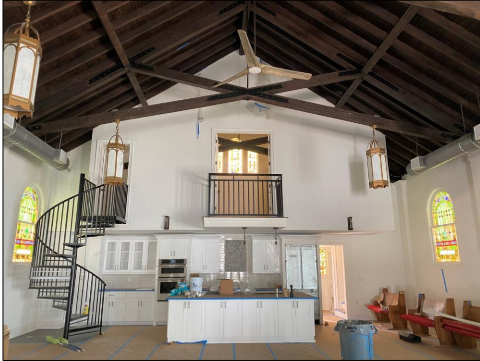
Figure 15: Adaptively reused sanctuary interior
