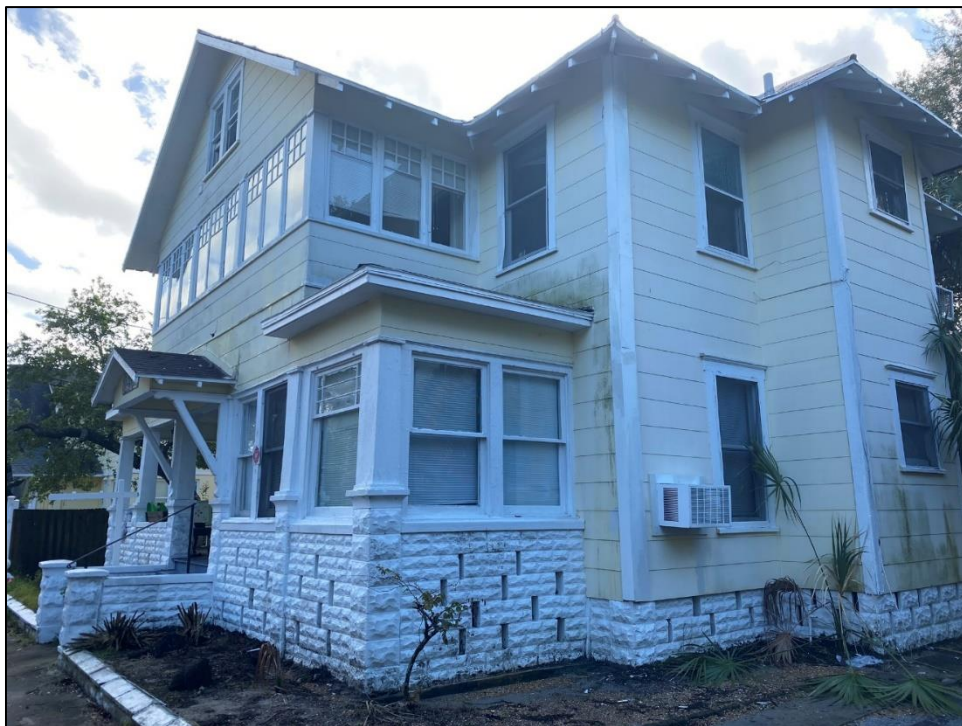
Figure 6: Façade and west elevation
