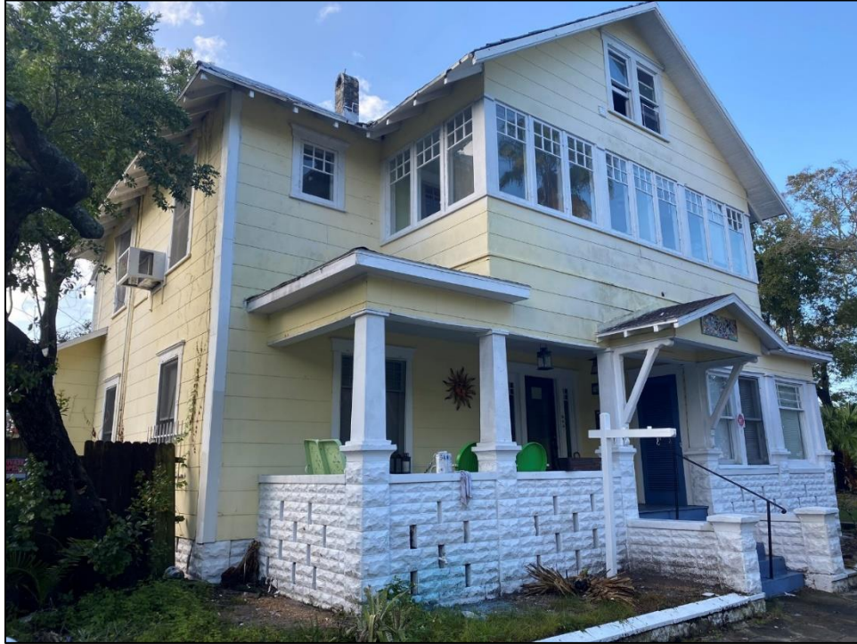
Figure 7: Façade and east elevation
