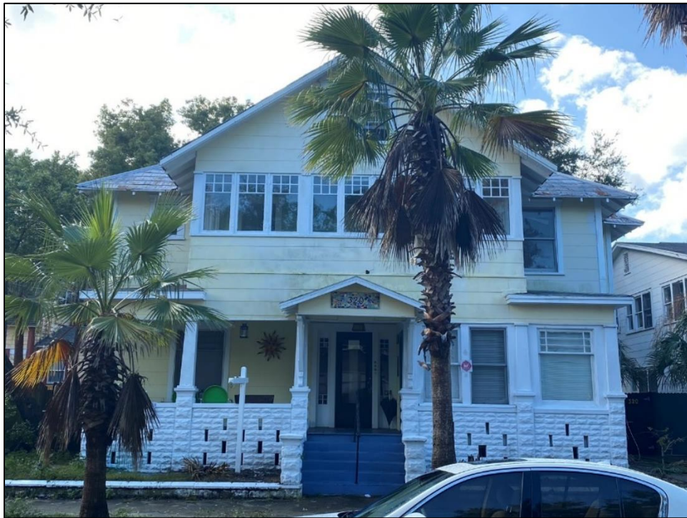
Figure 5: North façade of subject property
