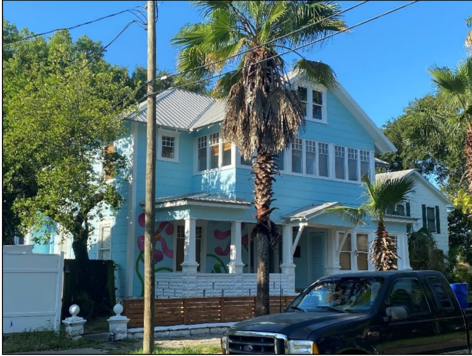
Figure 13: Façade and west elevation
