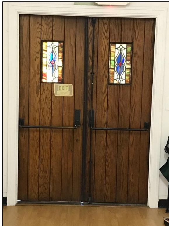
Figure 7: Doors at side entry to be reused
