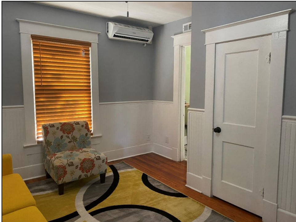
Figure 16: Rehabilitated living room with ductless mini split evaporator unit
