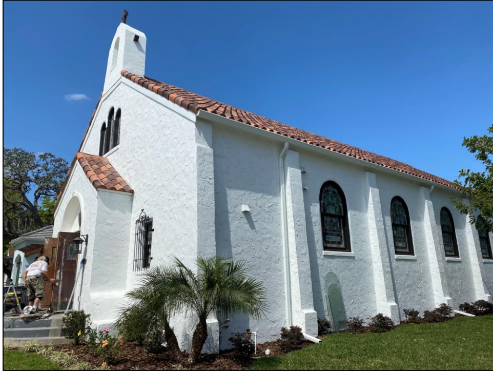
Figure 13: Façade and east elevation
