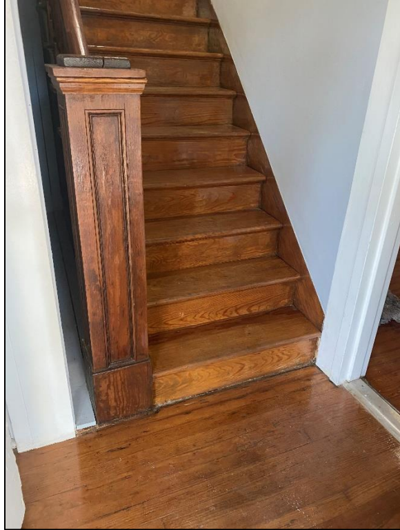
Figure 17: Restored stairs and newel post
