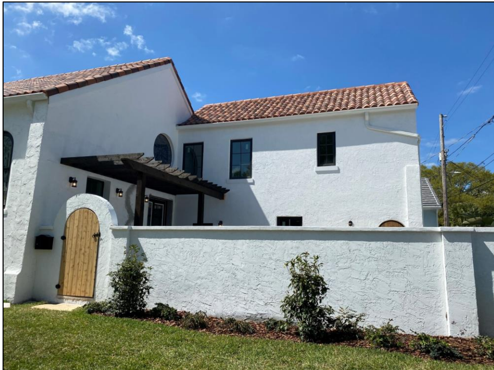
Figure 14: Addition from 8 th St N (east elevation)
