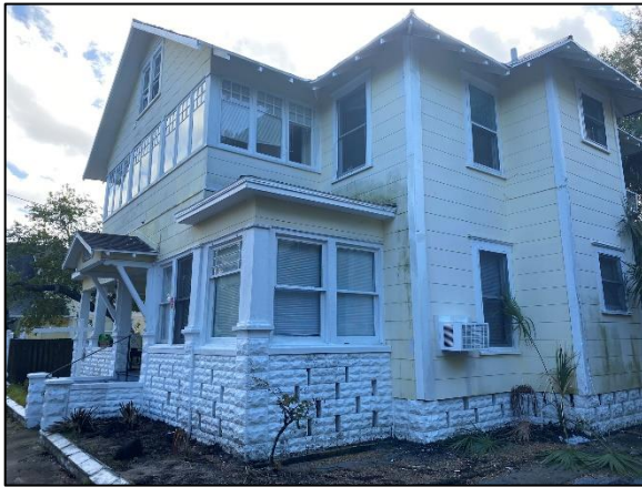
Figure 1: 320 6 th Ave N prior to rehabilitation
