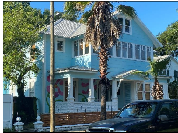
Figure 2: 320 6 th Ave N following rehabilitation
