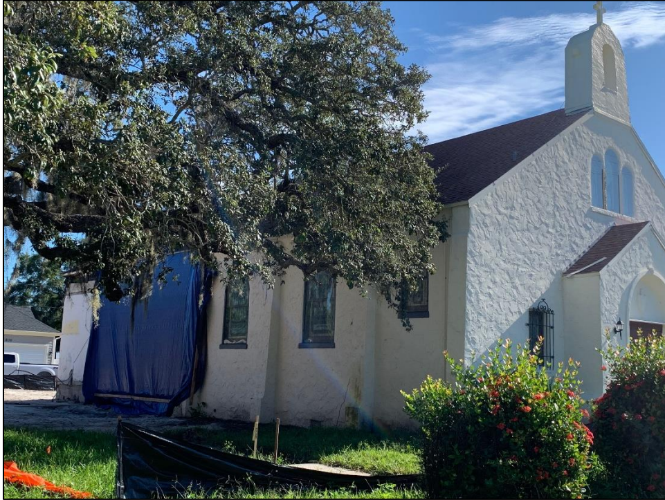
Figure 6: West elevation following demolition of non-historic addition
