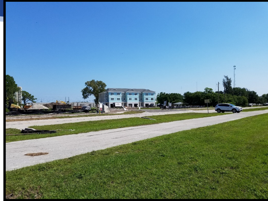
27 unit townhome development under construction to the east
