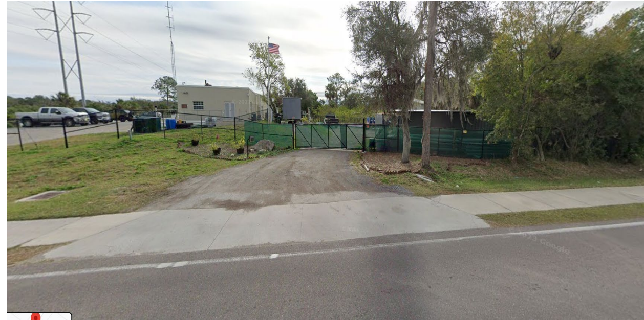
Looking southeast from Dixie Highway
